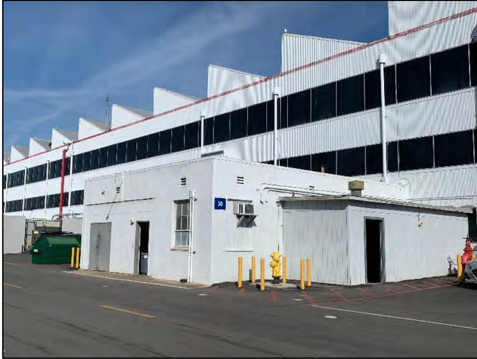
Figure 5.8-1 Building 30, Southwest and Southeast Façades View toward the north.
