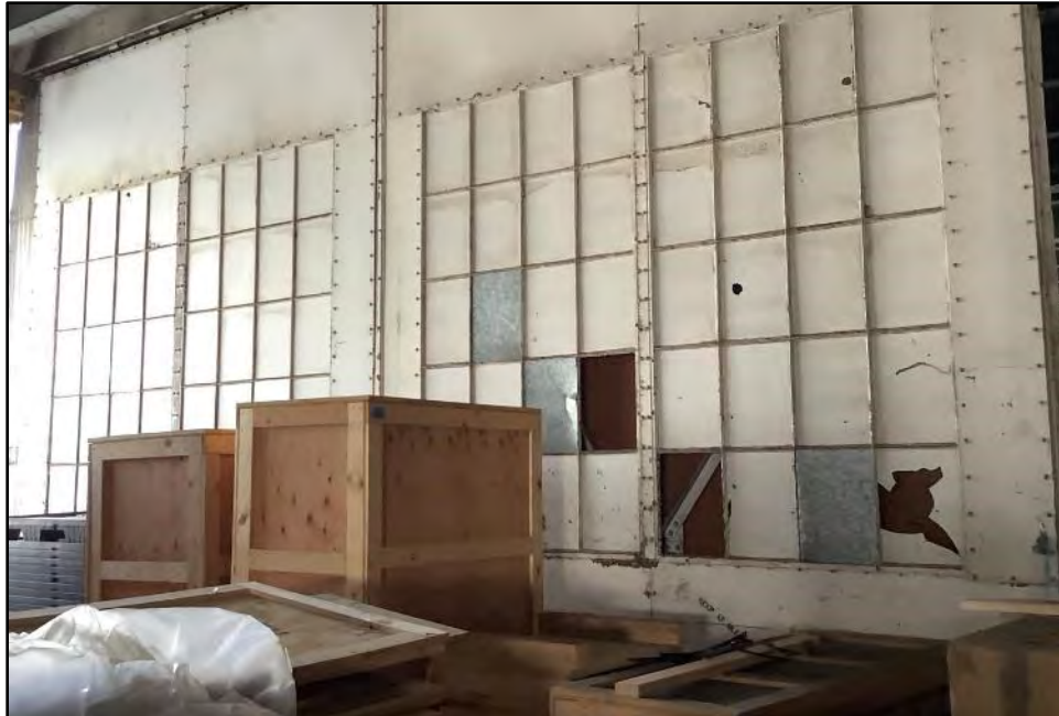
Figure 5.5-10 Building 8 Interior, Northeast Wall of Ground Floor View toward the east.
