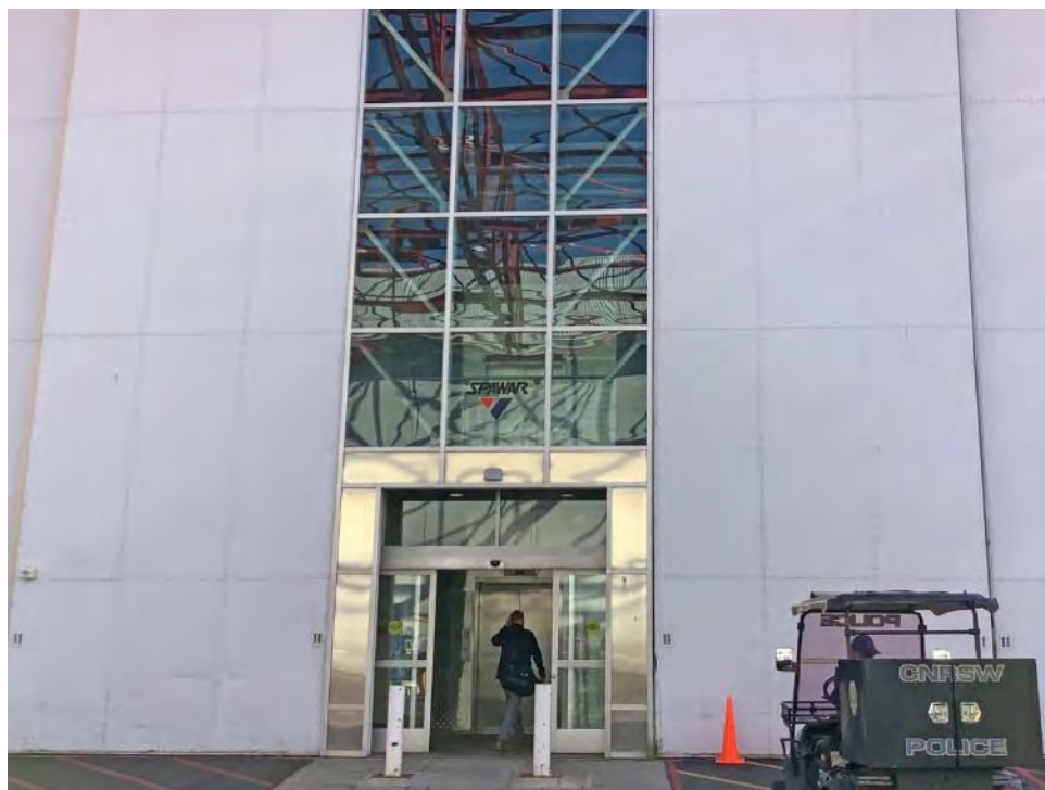
Figure 5.2-7 Building 1, New Entrance to Offices at Northwest Façade View toward the southeast.
