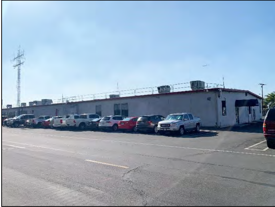
Figure 5.7-1 Building 28, Northwest and Northeast Façades View toward the south.
