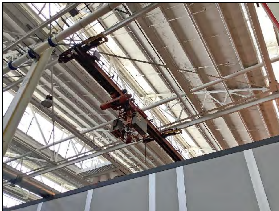
Image 4. Building 2, Crane Hoist. View toward the northeast.
