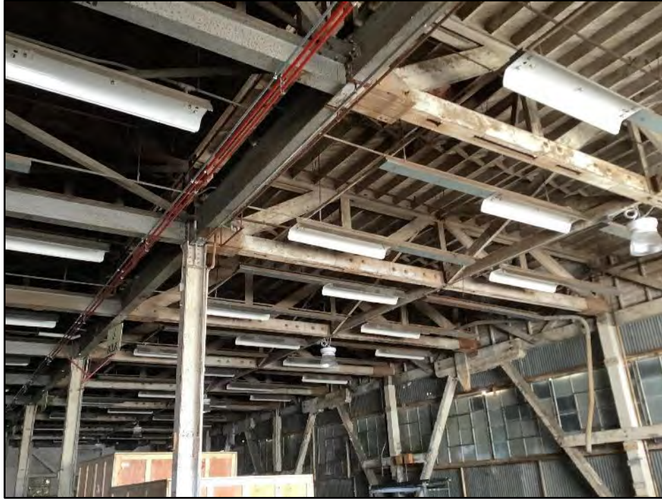
Figure 5.4-9 Building 7 Interior, View Toward the Northeast
