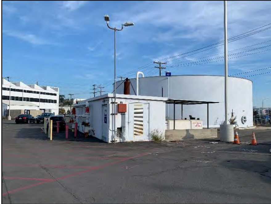
Figure 5.11-1 Tank 63 View toward the southeast.
