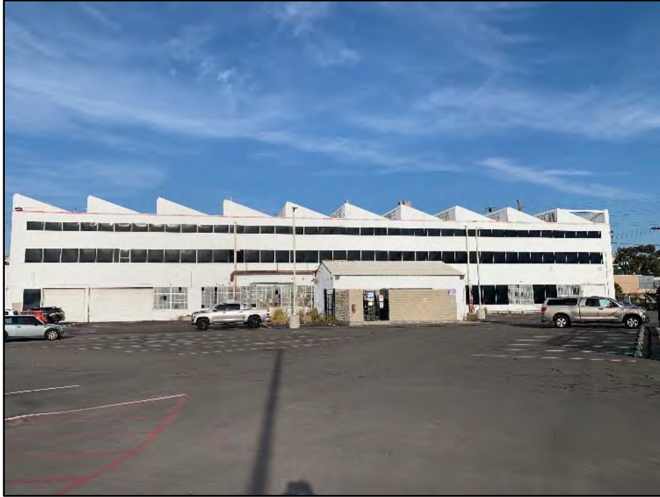
Figure 5.5-2 Building 8, Southeast End of Southwest Façade View toward the northeast.
