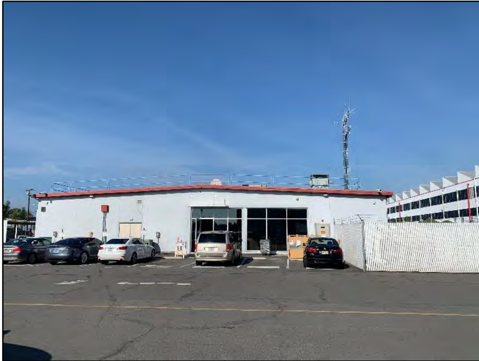
Figure 5.7-3 Building 28, Northwest Façade View toward the southeast.
