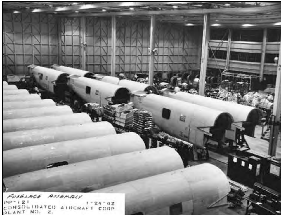
Figure 4.1-9 B-24 Fuselage Assembly at Plant 2 (January 24, 1942) Courtesy of San Diego Air and Space Museum.
