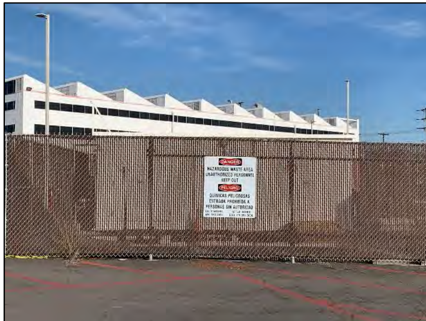
Figure 5.12-2 Building 73, South Façade View toward the north.
