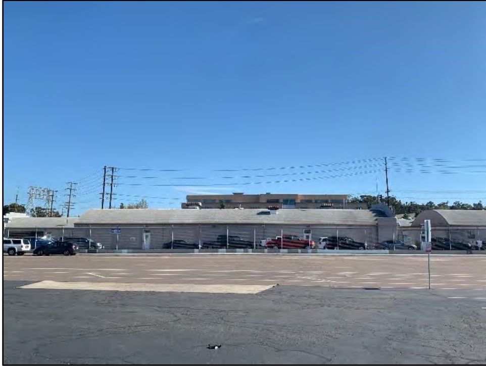
Figure 5.14-24 The West Façade of Building 3 View toward the east.
