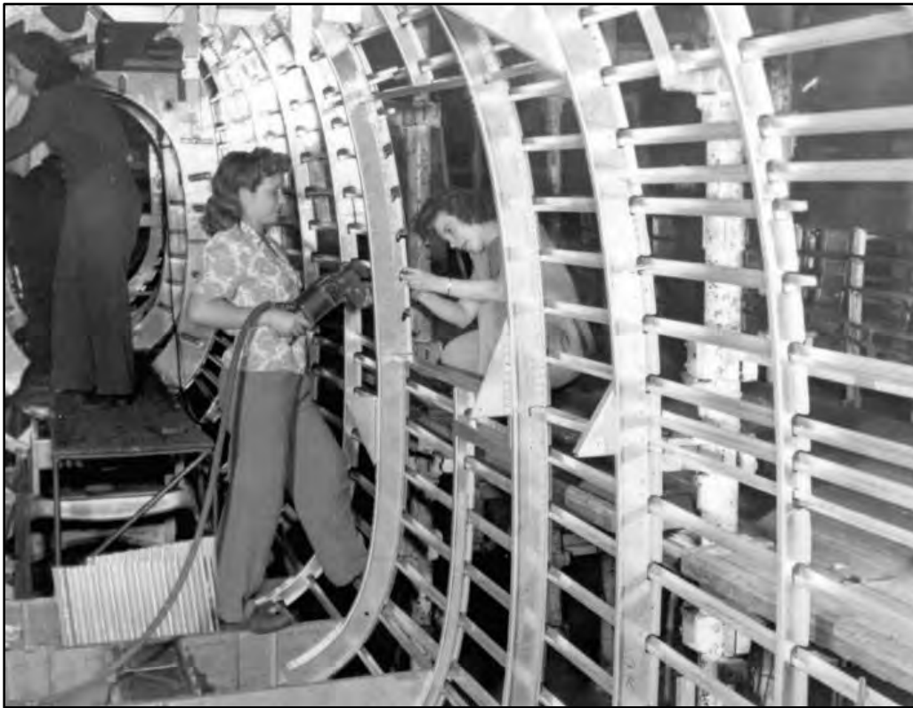
Figure 4.1-18 Women Assembling an Airframe, One with a Rivet Gun Courtesy of San Diego Air and Space Museum.
