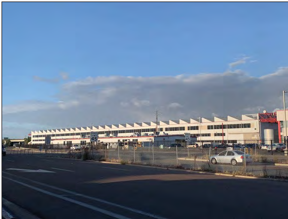
Image 7. Building 3, view toward the north.
