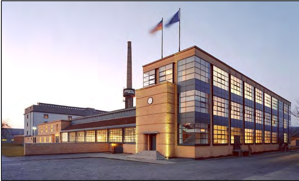
Figure 4.4-2 Fagus Factory, Alfeld, Germany, 1910
