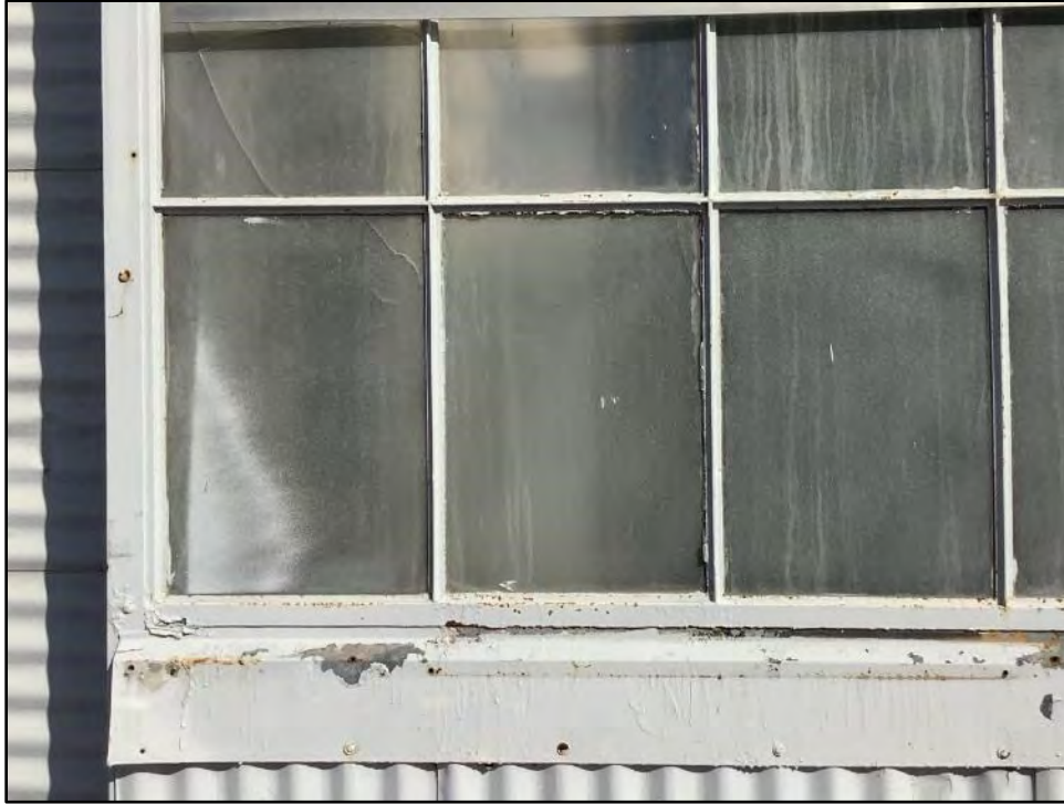
Figure 5.5-8 Building 8, Detail of Window at Southwest Façade View toward the northeast.
