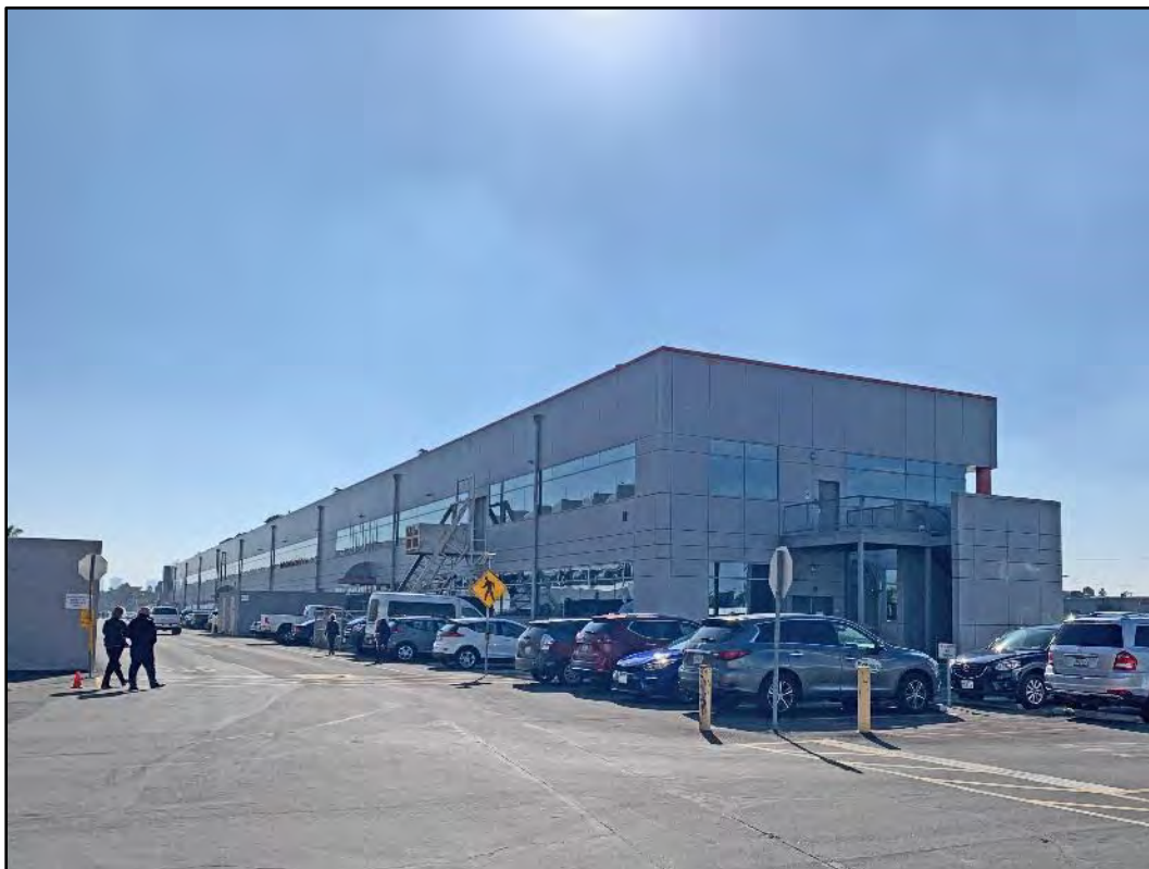
Figure 5.3-2 Building 4, Northwest and Northeast Façades View toward the south.
