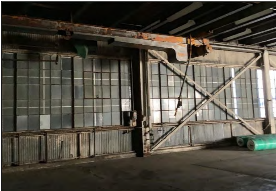
Figure 5.5-13 Building 8 Interior View toward the east.
