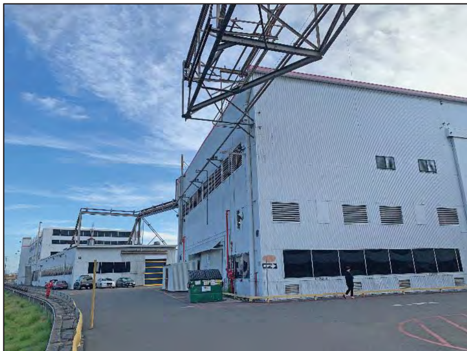
Image 3. Building 7, Northwest and Northeast Façades View toward the south.
