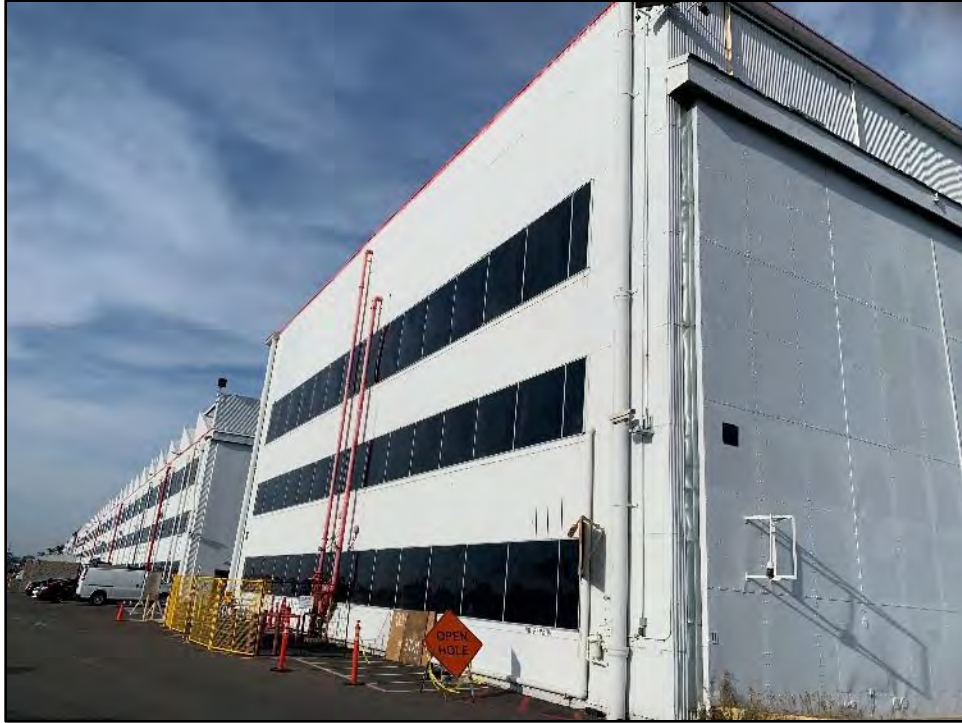
Figure 5.4-3 Building 7, Southwest Façade View toward the north.
