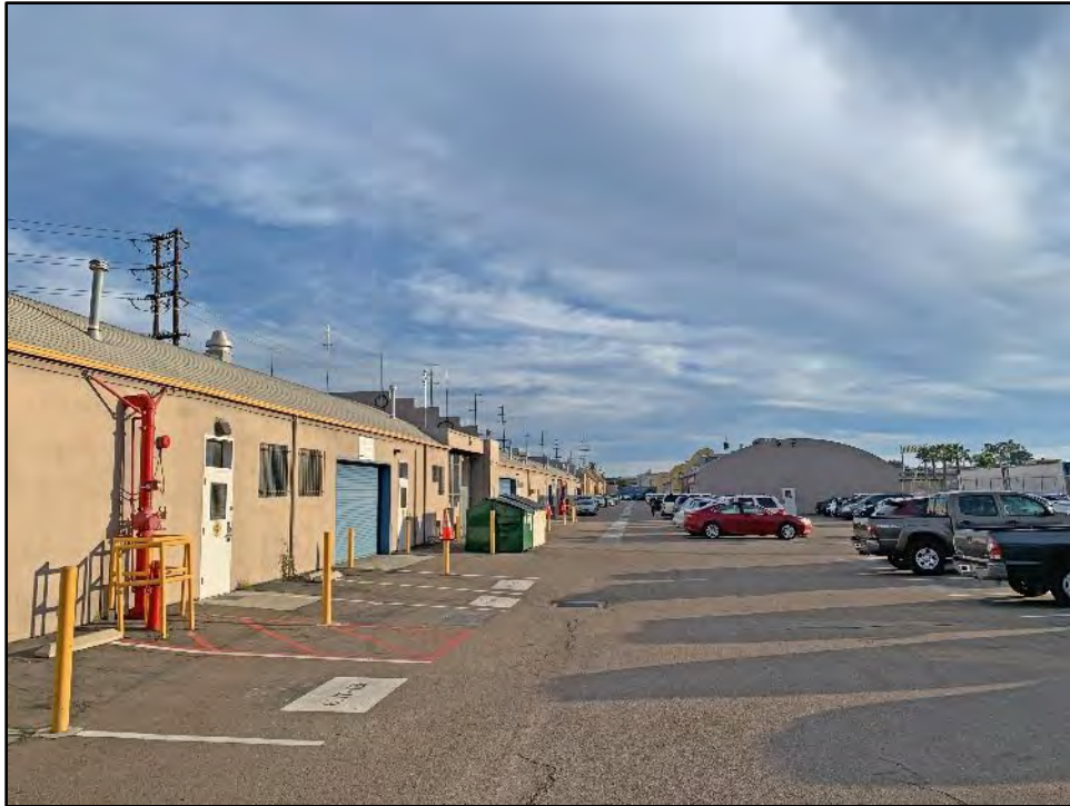
Figure 5.14-8 The West Façades of Buildings 4 and 2 and the North Façade of Building 3 View toward the southeast.
