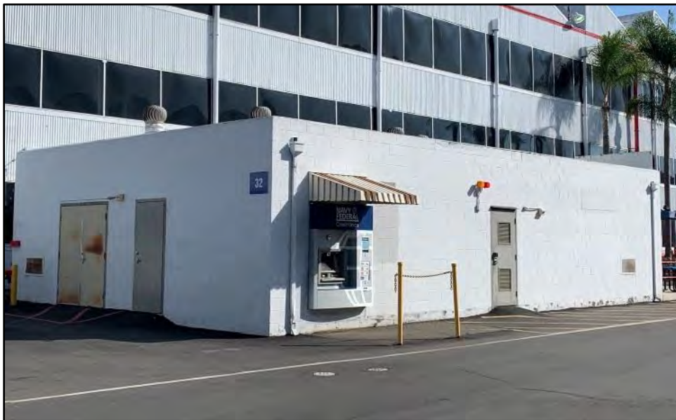
Figure 5.9-2 Building 32, Northwest and Southwest Façades View toward the east.
