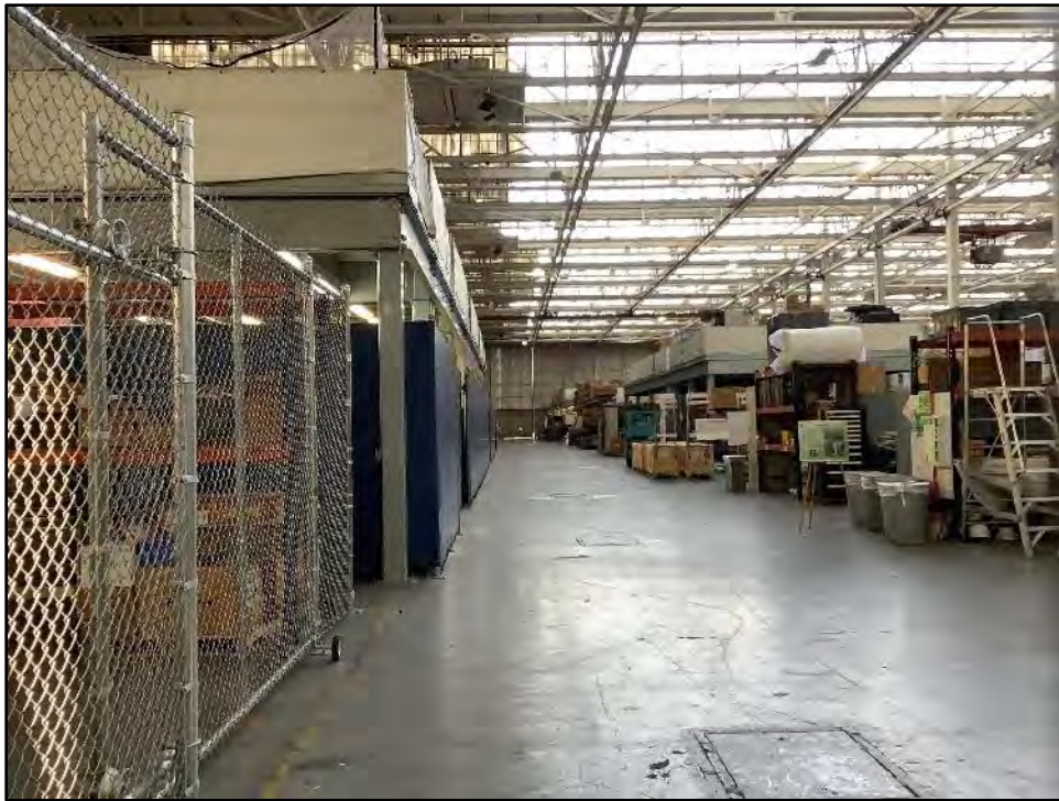
Figure 5.2-33 Building 2 Interior, Storage Areas on Ground Floor View toward the northwest.
