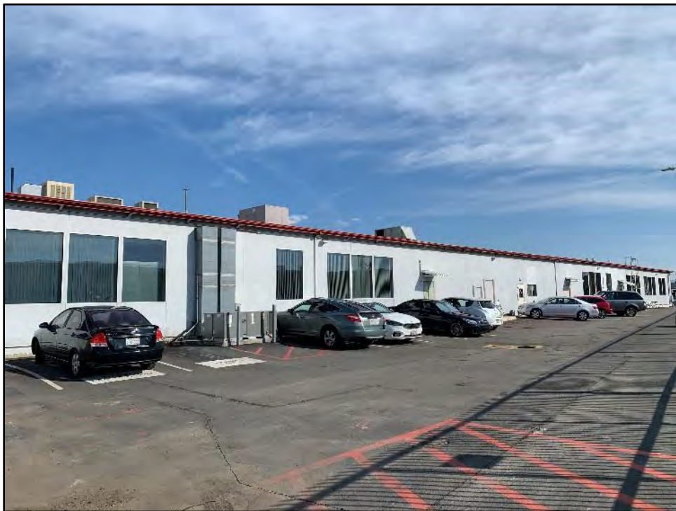
Figure 5.6-4 Building 27, Southwest Façade View toward the north.
