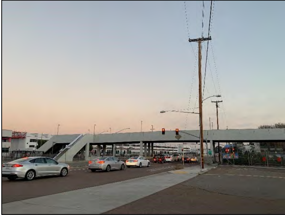
Figure 5.13-3 Northwest Side of the Bridge View toward the southeast.
