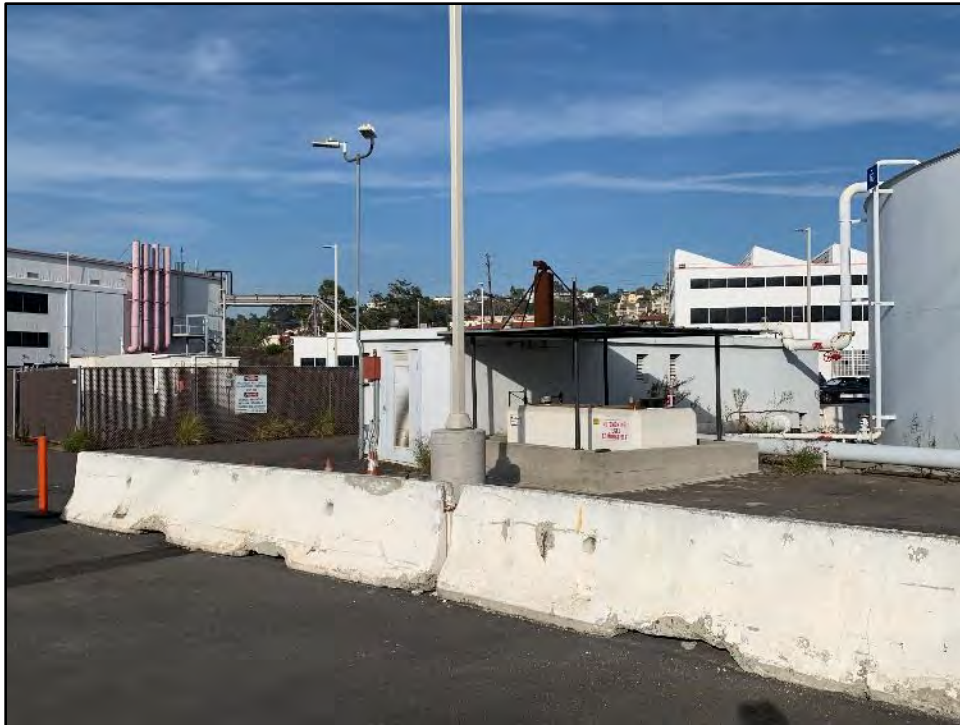
Figure 5.10-1 Building 37, the West and South Façades View toward the northeast.
