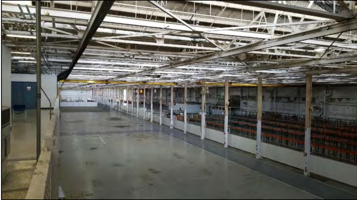
Figure 5.2-46 Building 3 Interior, Third Mezzanine View toward the southeast.
