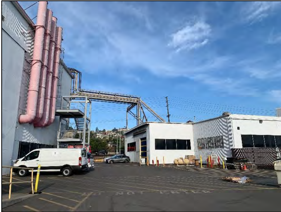
Figure 5.5-6 Building 7 (left) and Building 8 (right) View toward the northeast.
