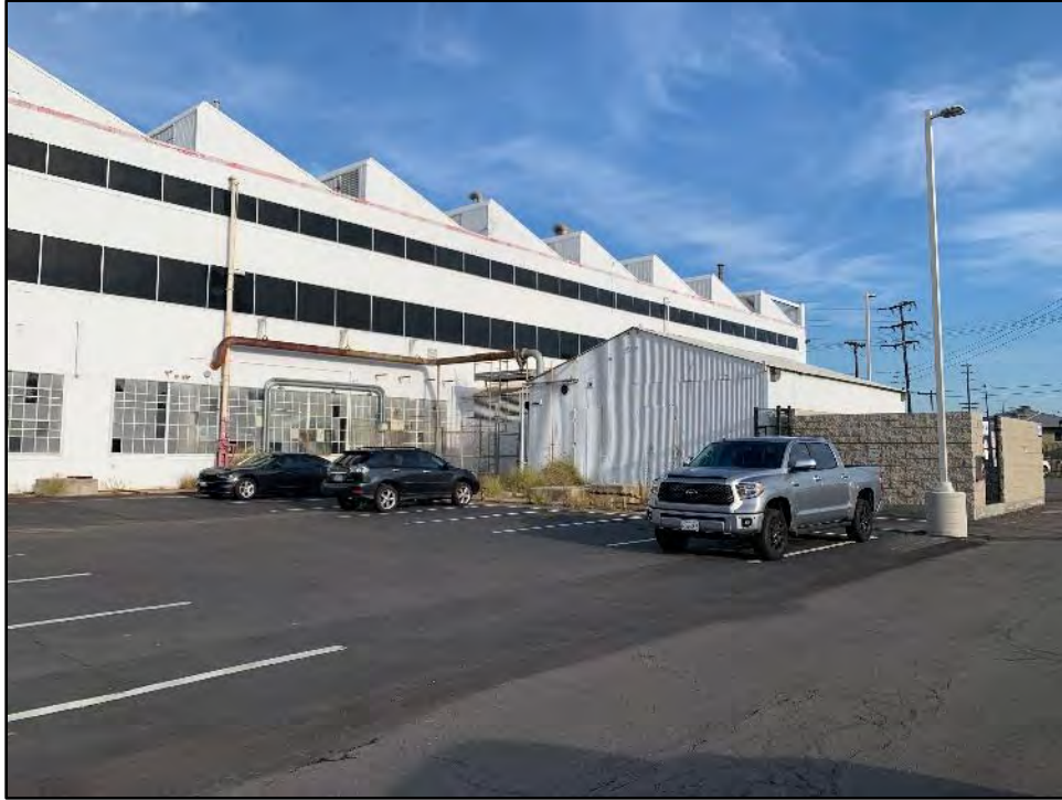
Figure 5.5-4 Building 8, Addition at Southwest Façade View toward the east.
