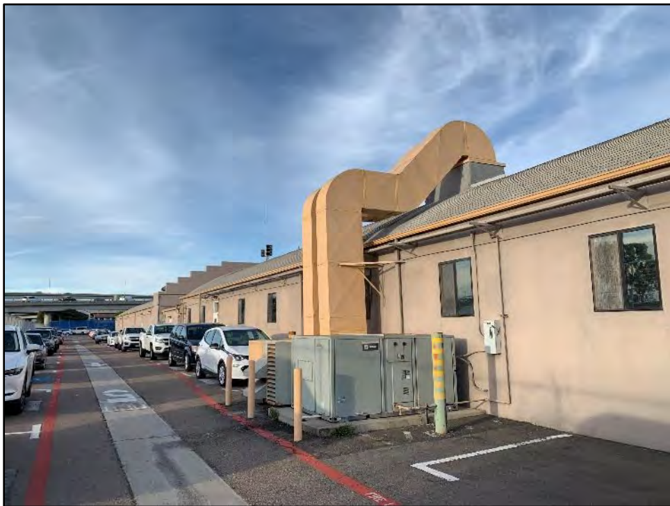
Figure 5.14-7 The West Façades of Buildings 3 and 1 View toward the northeast.
