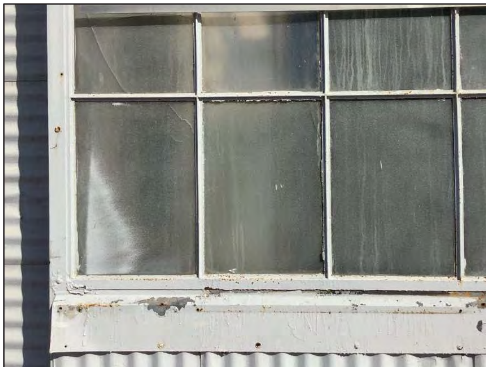
Image 7. Building 8, Detail of Window at Southwest Façade. View toward the northeast.
