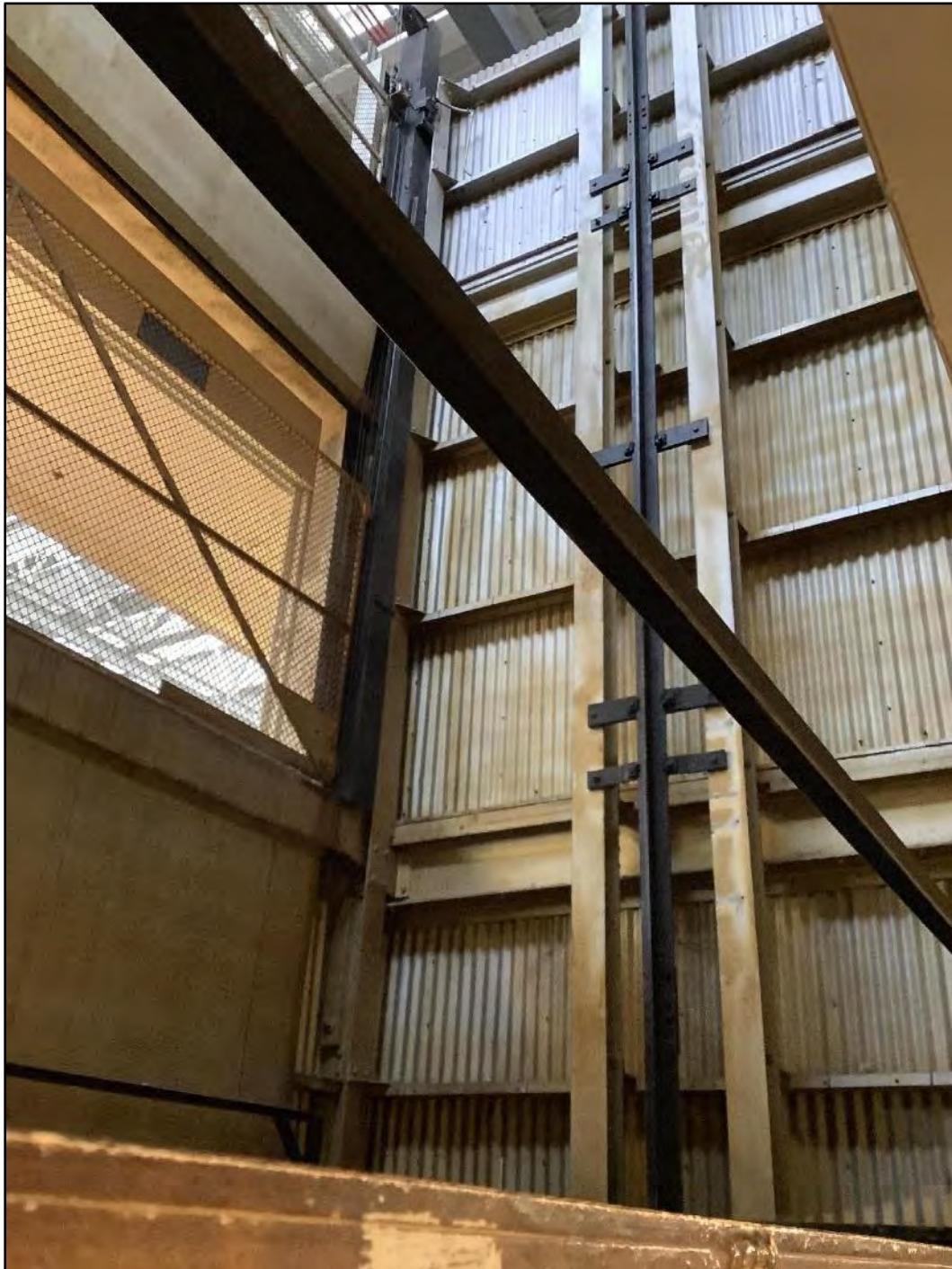
Figure 5.2-21 Building 1 Interior, Freight Elevator View toward the southeast.
