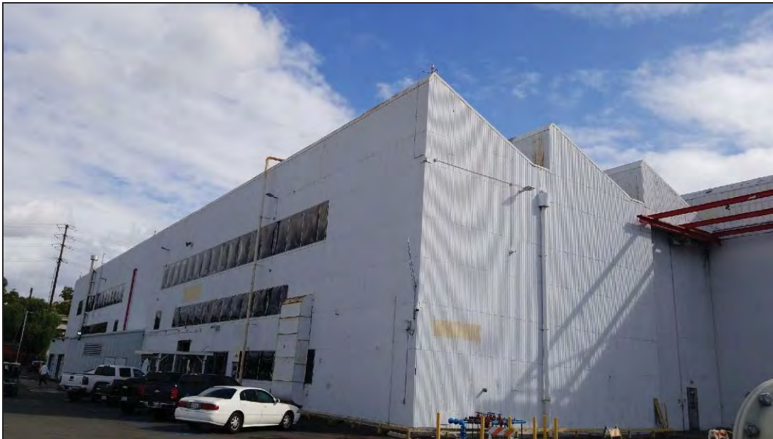
Image 5. Building 7, view toward the east.
