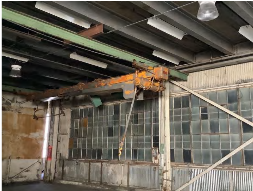
Figure 5.5-11 Building 8 Interior, Ground Floor View toward the north.
