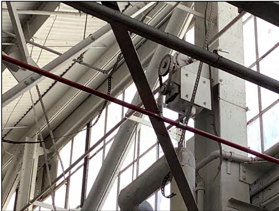
Figure 5.2-11 Building 1 Interior, Detail of Window Operating Mechanisms View toward the west.
