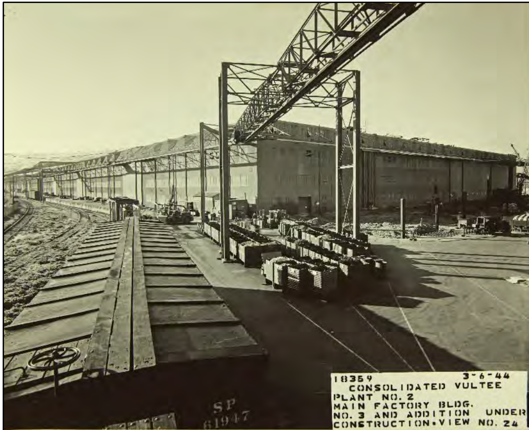
Figure 5.2-1 Historical Photo of the Crane Monorail
