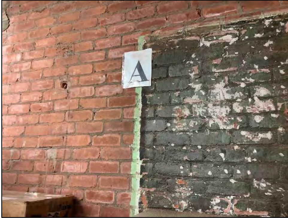
Figure 5.14-50 Detail of Brick Wall in Building 4 View toward the south.
