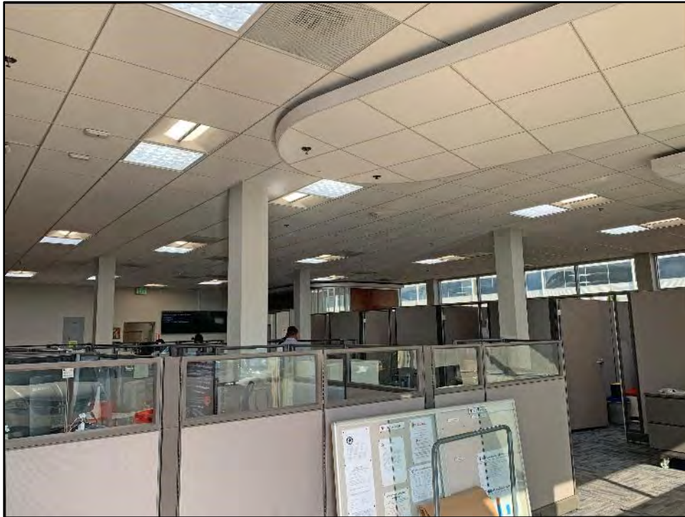
Figure 5.7-5 Building 28 Interior View toward the north from the southeast entrance.
