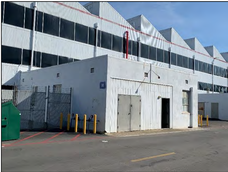
Figure 5.8-2 Building 30, the Northwest and Southwest Façades View toward the east.
