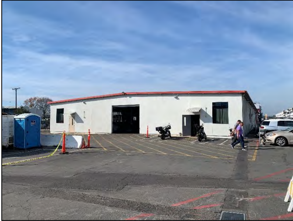
Figure 5.6-3 Building 27, Southeast Façade View toward the northwest.
