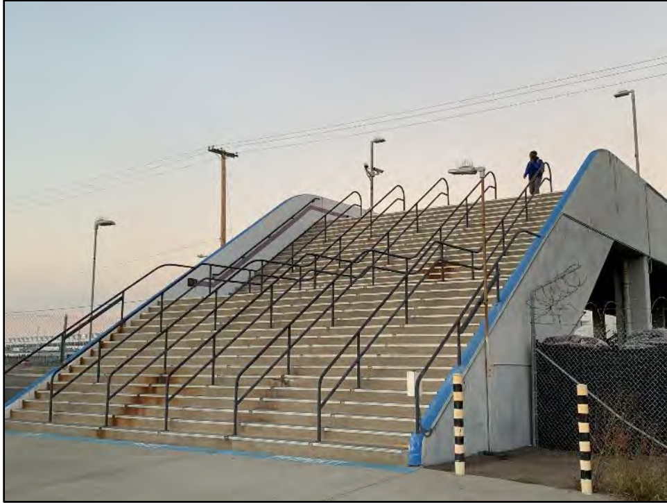
Figure 5.13-5 The Southwest Side of the Bridge View toward the northeast.
