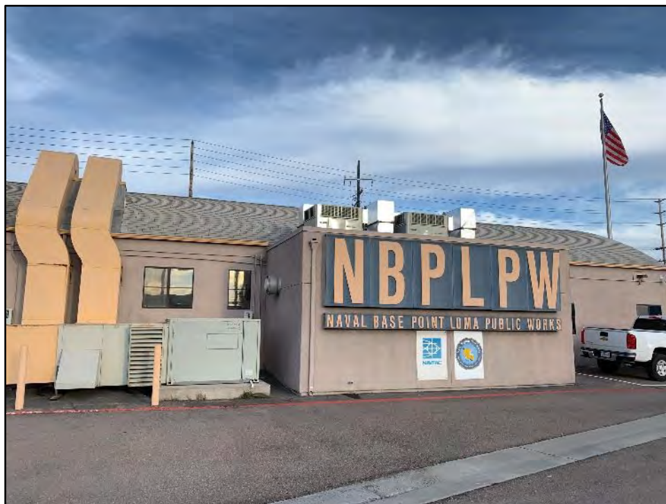
Figure 5.14-17 Detail of the West Façade of Building 1 South View toward the east.
