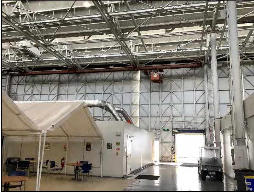
Figure 5.2-14 Building 1 Interior, Crew-operated Cab and Hangar-type Doors View toward the southeast.
