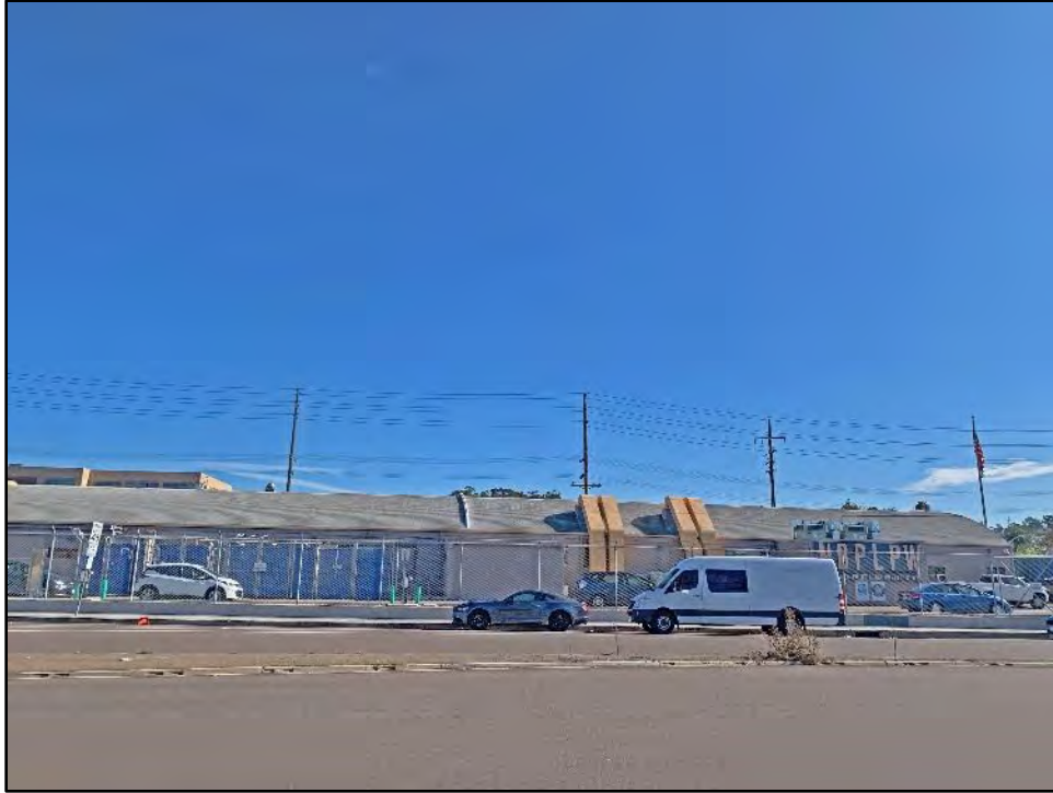
Figure 5.14-14 The West Façade of Building 1 View toward the east.
