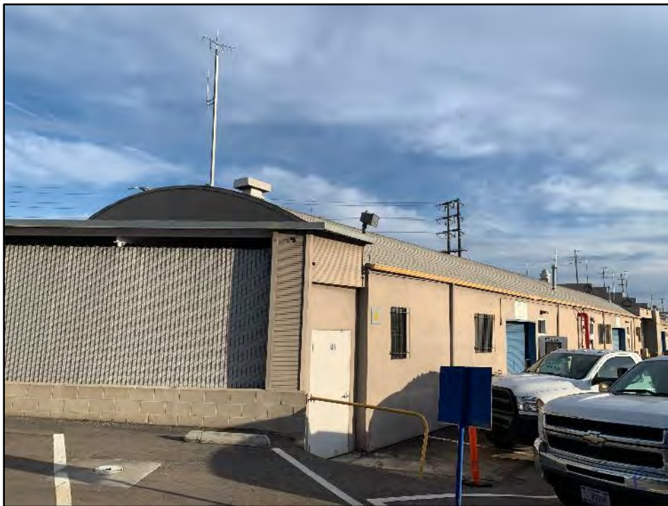
Figure 5.14-25 The North and West Façades of Building 4 View toward the southeast.
