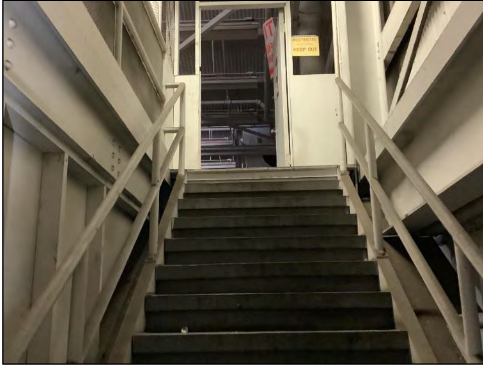
Figure 5.5-16 Building 8 Interior, Stairway to Third Floor View toward the southeast.
