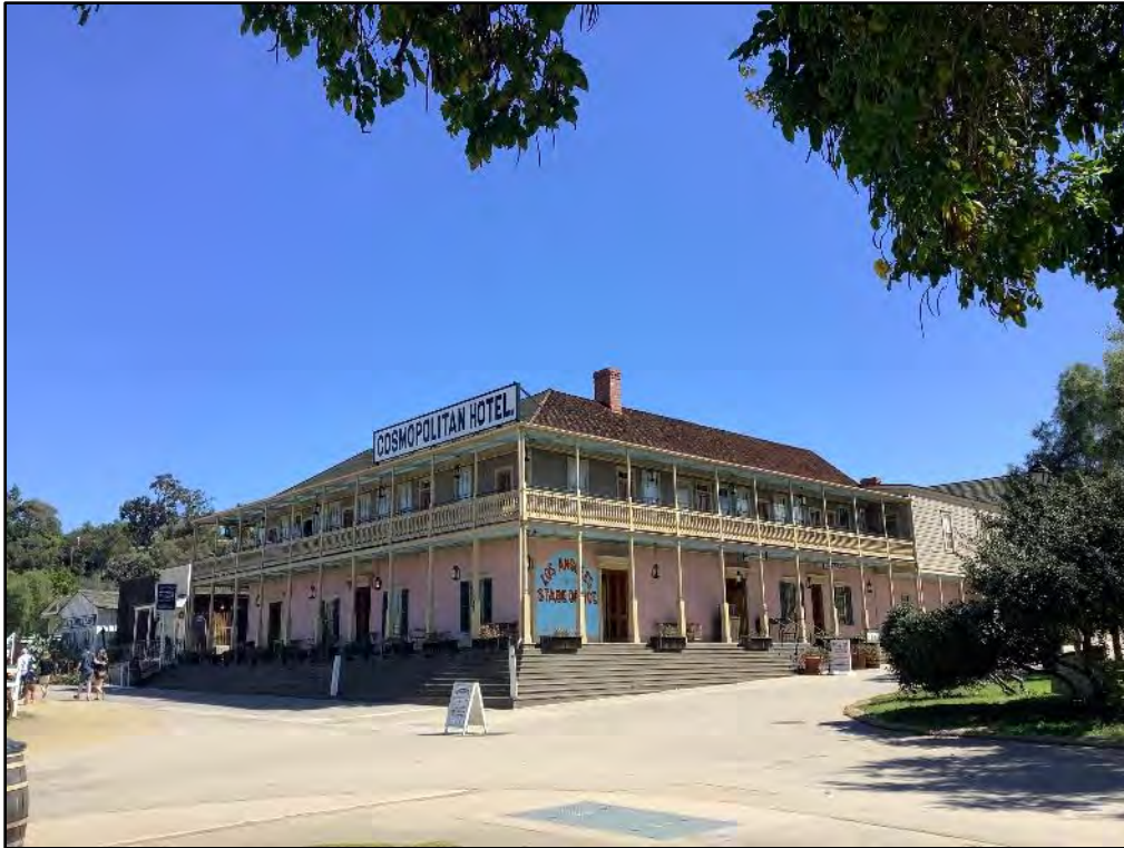
Figure 5.2-6 Casa de Bandini at 2660 Calhoun Avenue, looking Northeast
