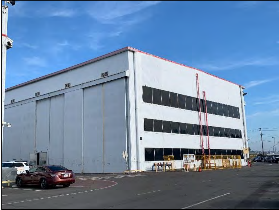
Figure 5.4-1 Building 7, Northwest and Southwest Façades View toward the east.
