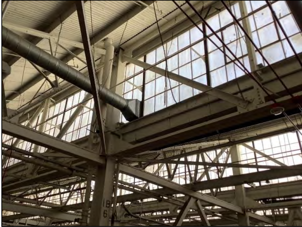
Figure 5.2-10 Building 1 Interior, Detail View of Sawtooth Window Arrangements View toward the northwest.
