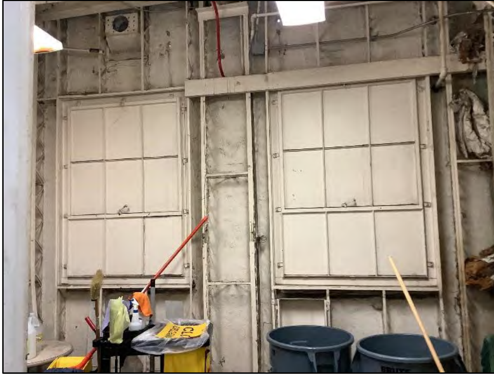
Figure 5.8-4 Building 30, Original Steel Windows from the Interior View toward the northwest.
