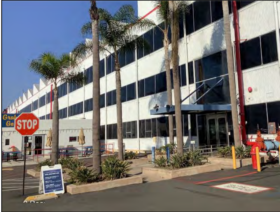
Image 2. Building 2, Southwest Façade. View toward the north.
