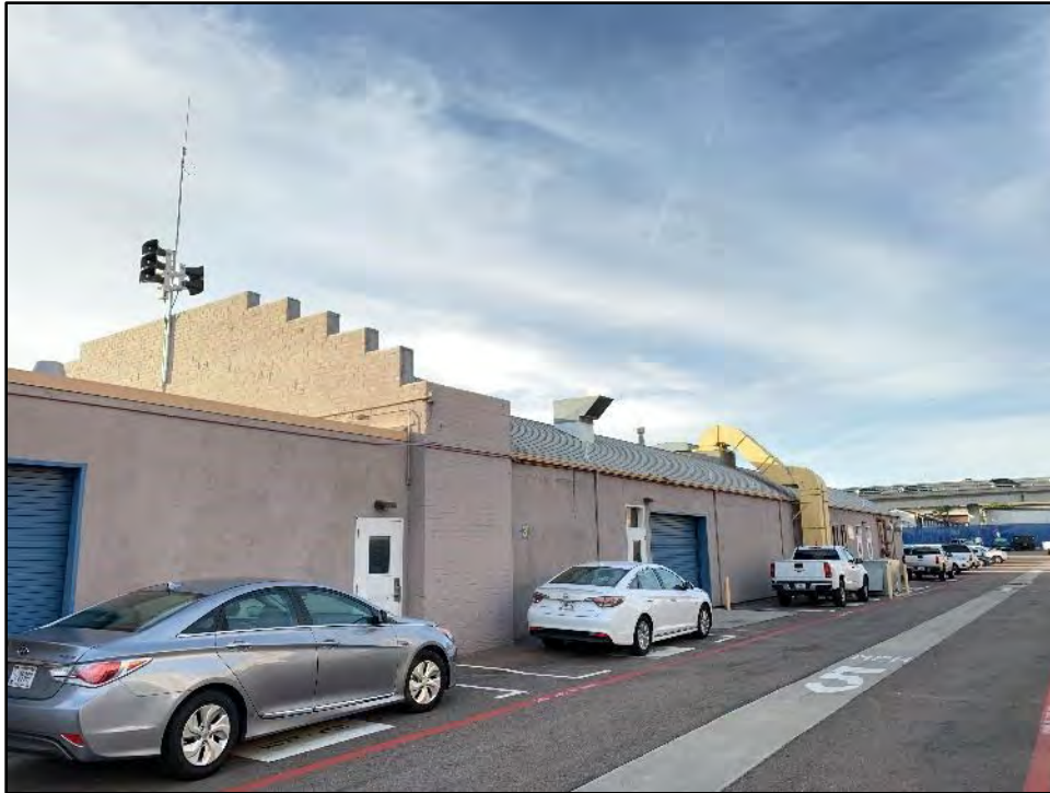
Figure 5.14-22 The East Façade of Building 3 View toward the northwest.
