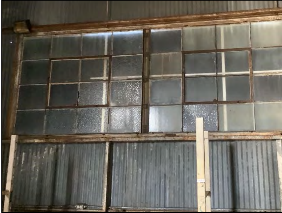
Figure 5.5-12 Building 8 Interior View toward the northeast.
