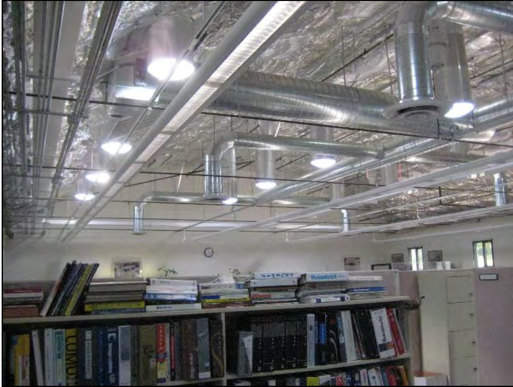
Figure 5.14-52 Ceiling of Remodeled Section of Building 4, Showing Insulation and Skylights
