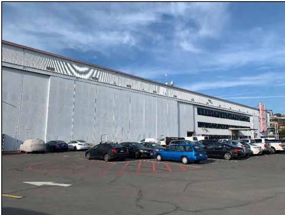
Figure 5.4-2 Building 7, Southeast Façade View toward the north.
