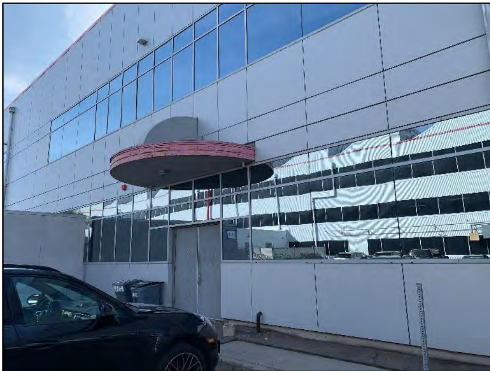
Figure 5.3-10 Building 4, Original Canopy at Northeast Façade View toward the south.
