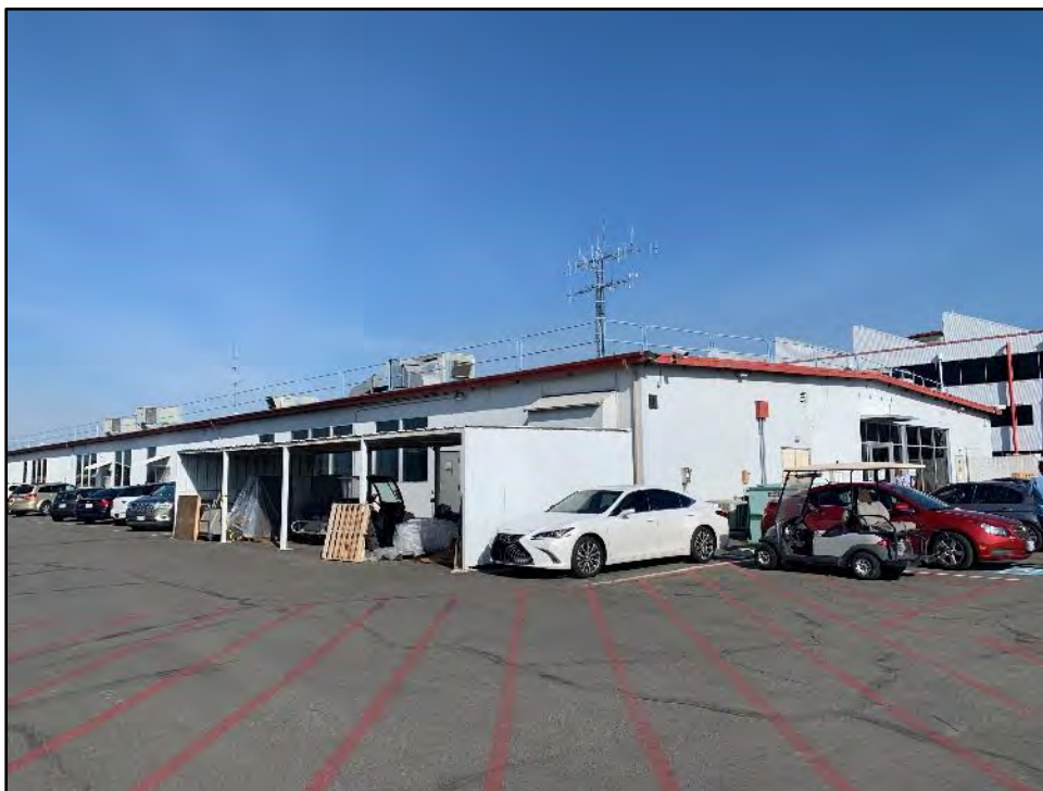
Figure 5.7-4 Building 28, Southwest and Southeast Façades View toward the north.
