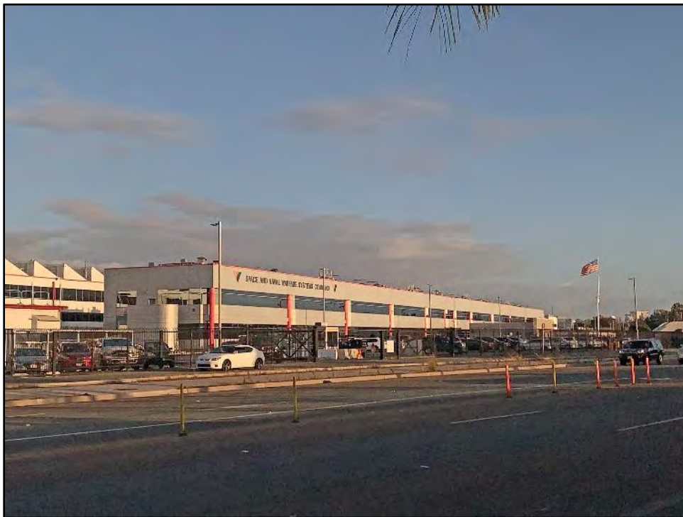
Figure 5.3-4 Building 4, Northwest and Southwest Façades View toward the southeast.
