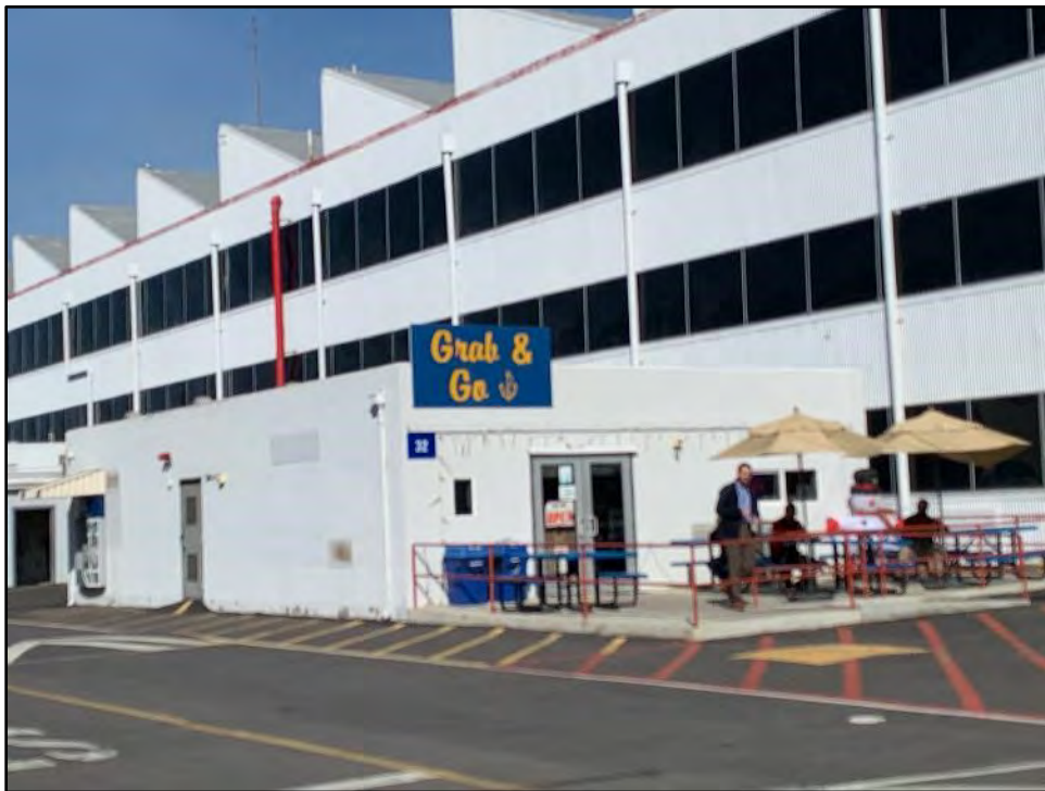
Figure 5.9-4 Building 32, Southwest and Southeast Façades View toward the north.
