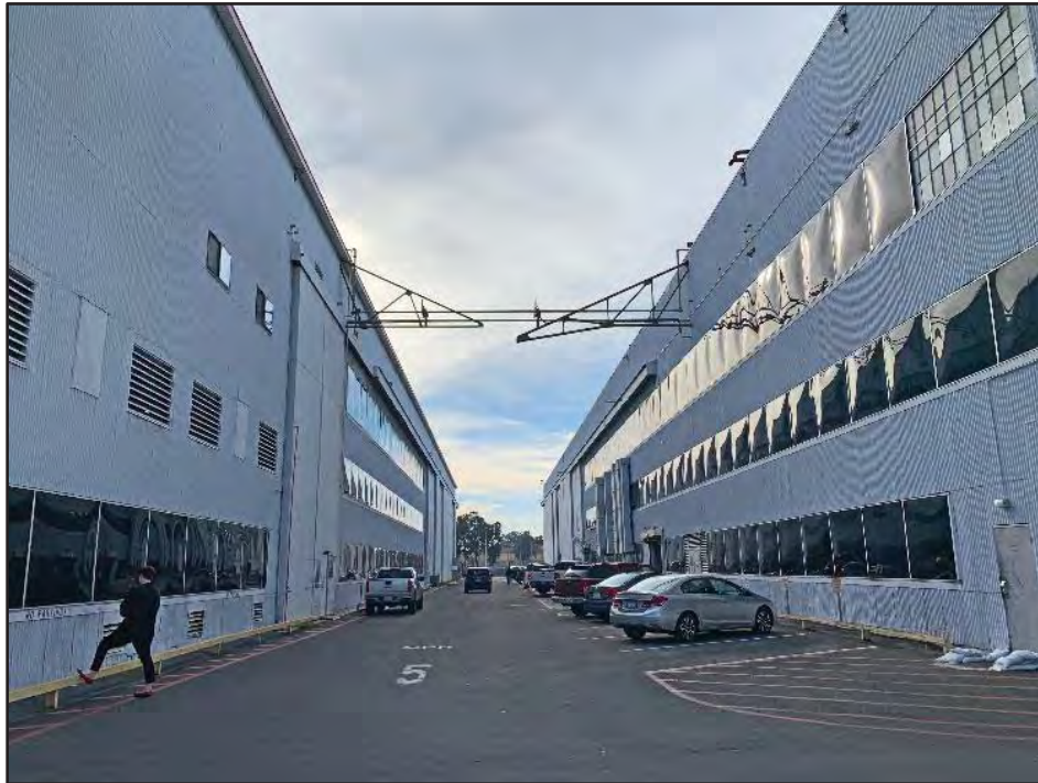
Image 1. Northwest Façade (right) and Building 7, Southeast Façade (left). View toward the southwest.
