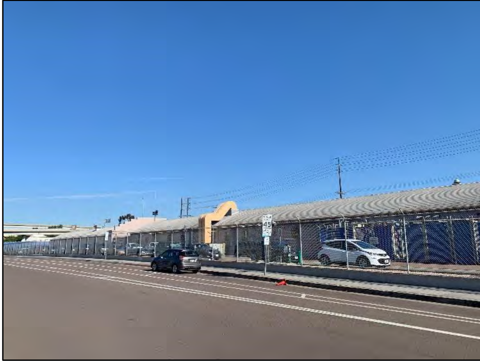
Figure 5.14-6 The West Façades of Buildings 3 and 1 View toward the northeast.
