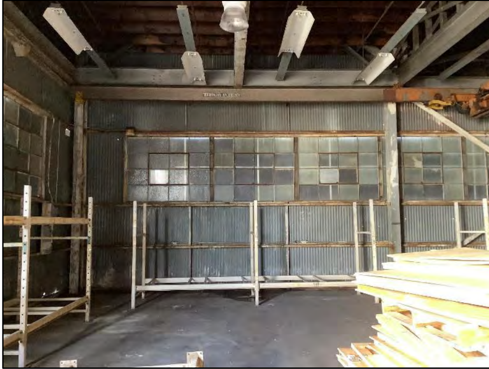
Figure 5.5-14 The American Monorail Tag on a Crane Rail at the Northeast Side of Building 8 View toward the northeast.
