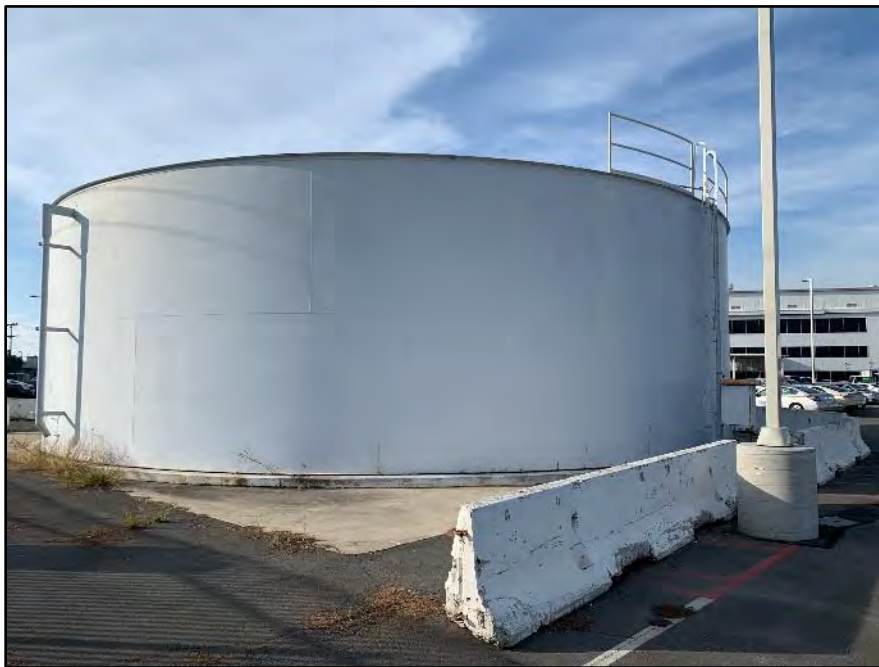
Figure 5.11-2 Tank 63 View toward the northeast.
