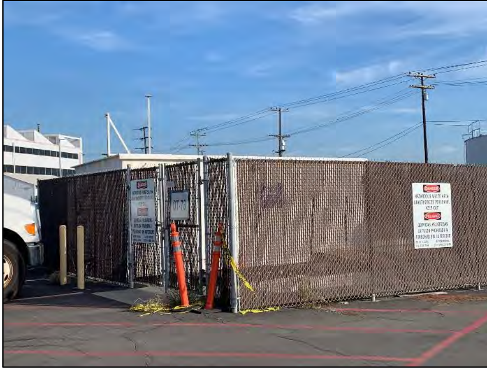
Figure 5.12-3 Building 73, North and West Façades View toward the southeast.
