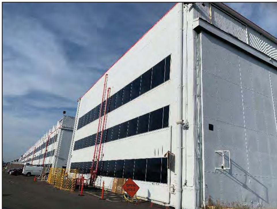
Image 2. Building 7, Southwest Façade. View toward the north.
