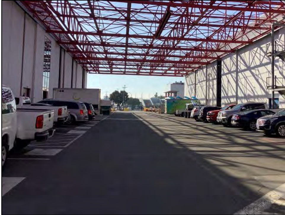
Figure 5.2-6 Building 1, Northwest Façade (left) and Building 2, Southeast Façade (right) View toward the west.
