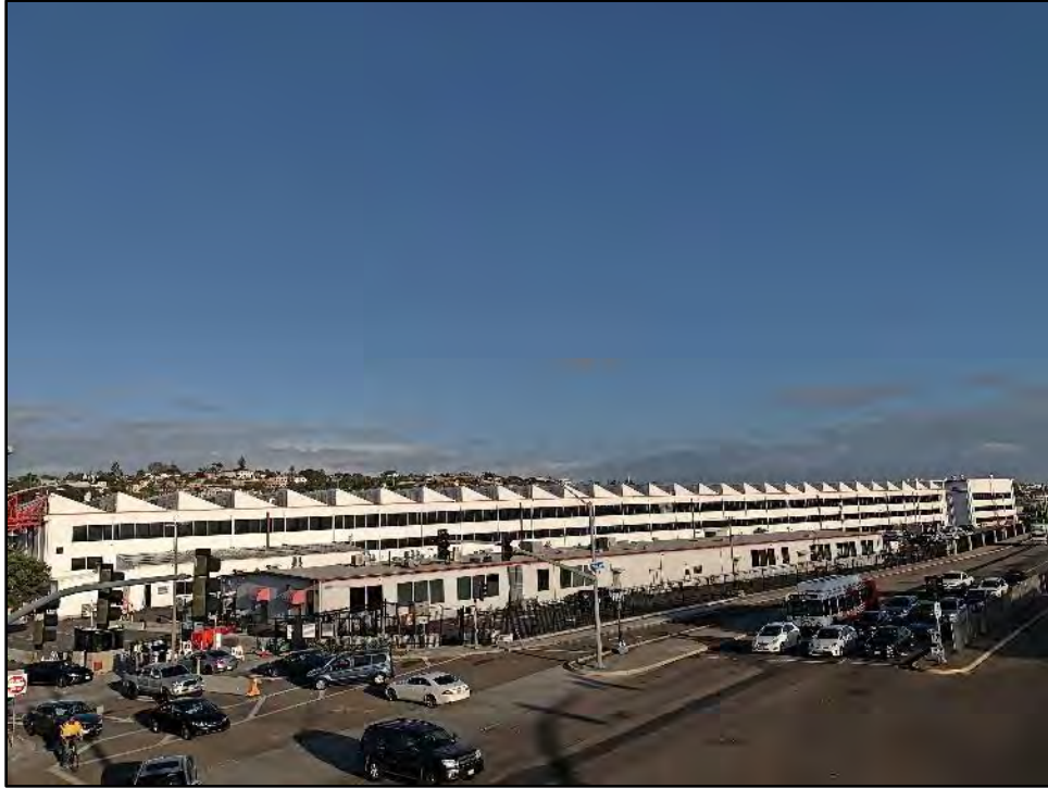
Figure 5.2-4 Building 1, Southwest Façade View toward the southeast.
