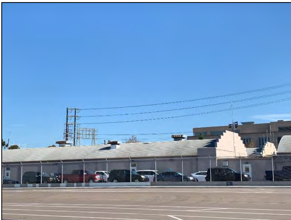
Figure 5.14-9 Overview of the Complex toward the Northeast
