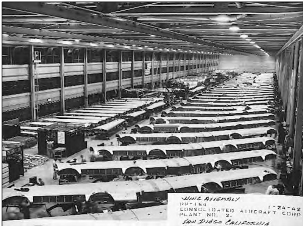
Figure 4.1-7 B-24 Wing Assembly at Plant 2 (January 24, 1942) Courtesy of San Diego Air and Space Museum.
