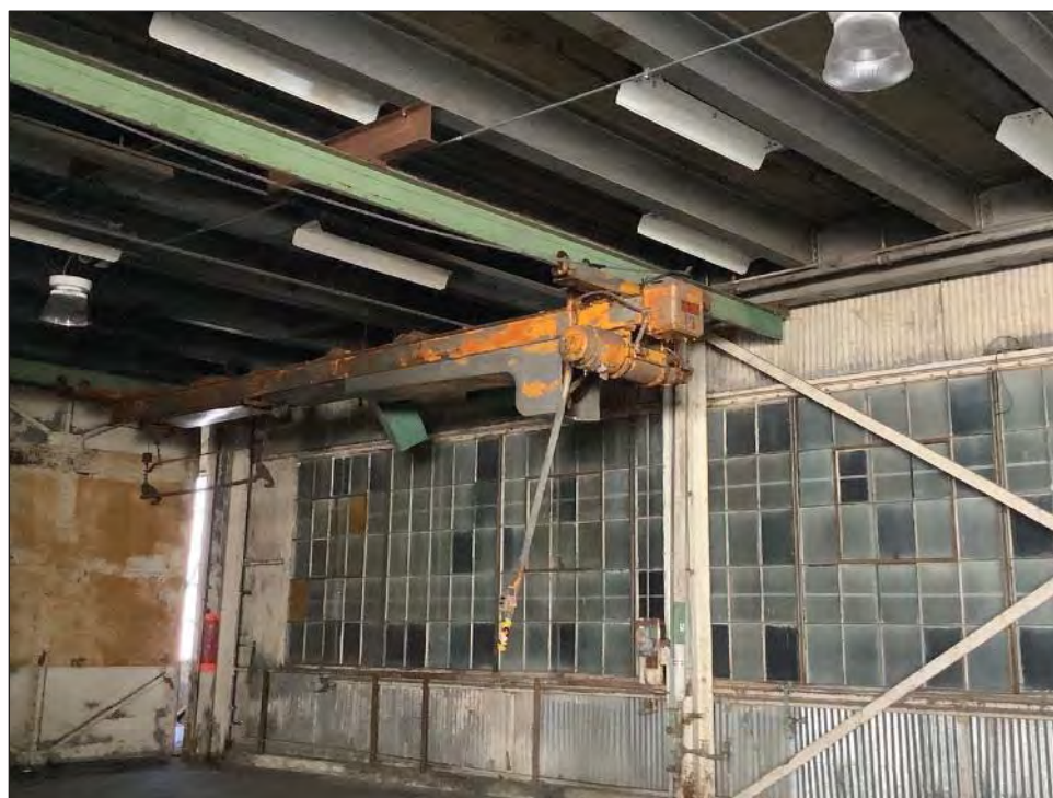
Image 9. Building 8 Interior, Ground Floor. View toward the north.
