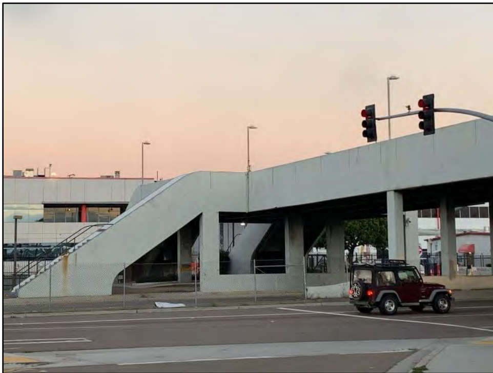
Figure 5.13-4 Northwest Side of the Bridge and Side Steps View toward the east.
