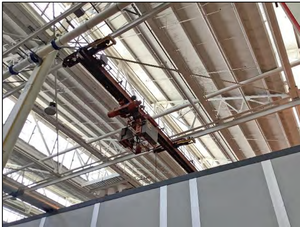
Figure 5.2-29 Building 2, Crane Hoist View toward the northeast.
