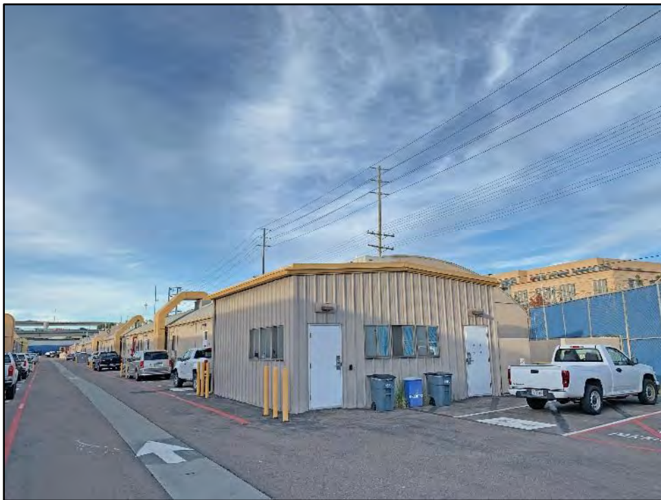
Figure 5.14-21 The West and South Façades of Building 2 View toward the northeast.
