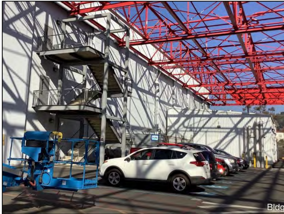
Figure 5.2-28 Building 2, Exterior Stairs and Addition at the Southeast Façade View toward the north.
