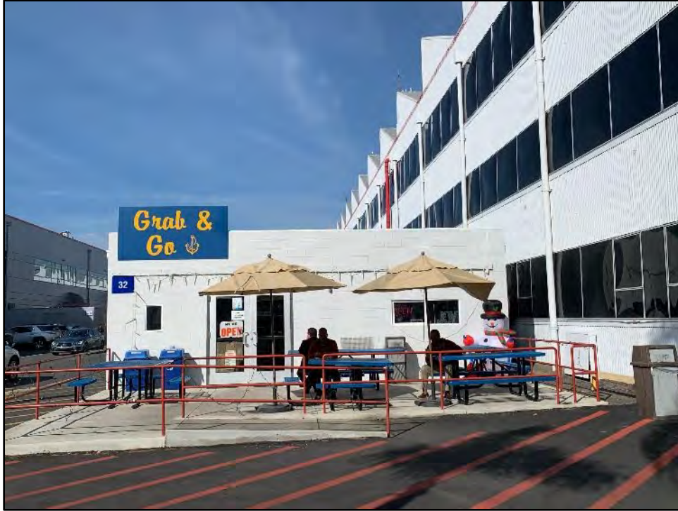
Figure 5.9-1 Building 32, the Primary (Southeast) Façade View toward the northwest.
