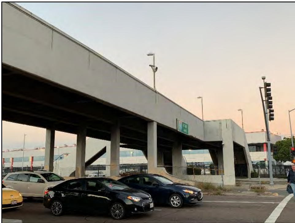
Figure 5.13-6 The Southeast Side of the Bridge View toward the northeast.
