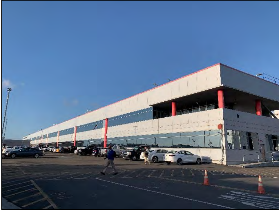
Figure 5.3-3 Building 4, Southwest and Southeast Façades View toward the north.
