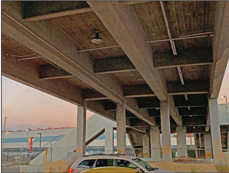
Image 3. Detail of the Underside of the Deck. View toward the east.
