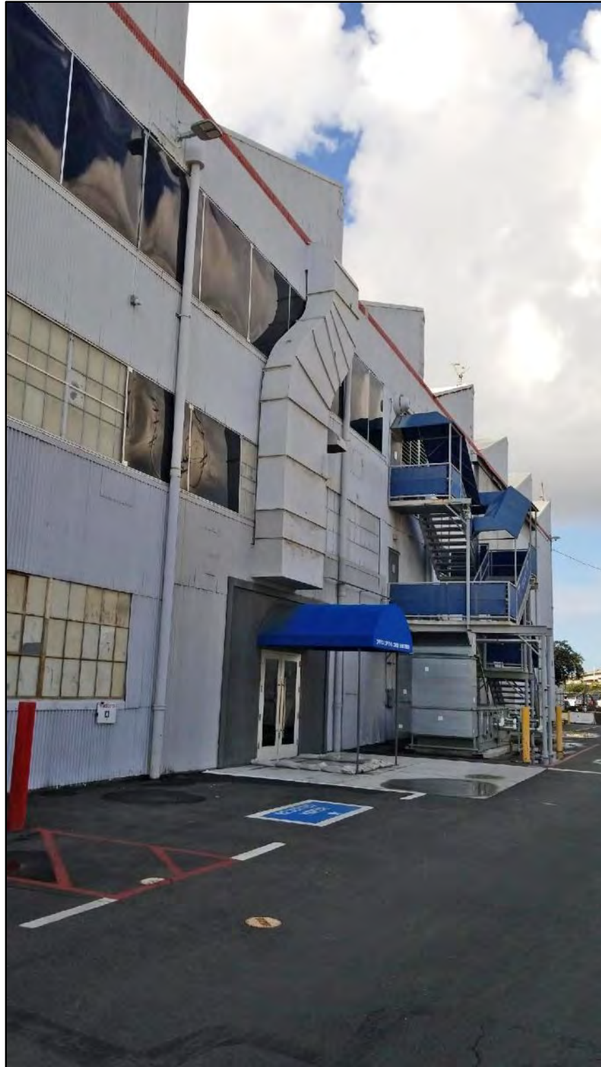
Figure 5.2-43 Building 3, Entrance and Stairway Addition at the North End of the Northeast Façade View toward the north.
