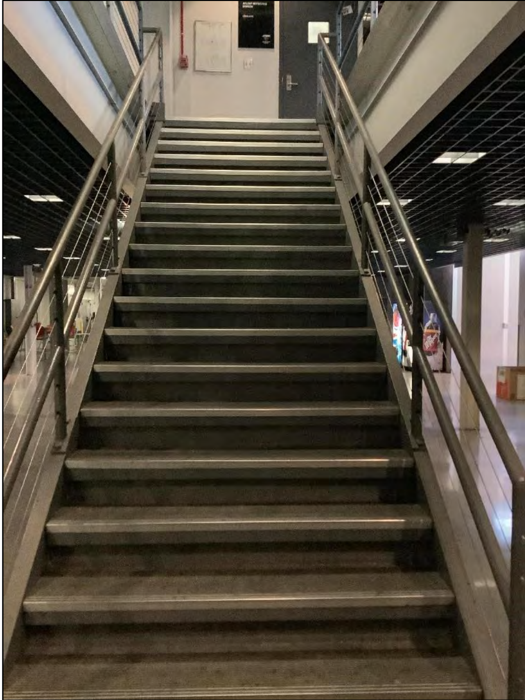
Figure 5.2-37 Building 2 Interior, Stairway to the Second Floor Mezzanine View toward the northwest.
