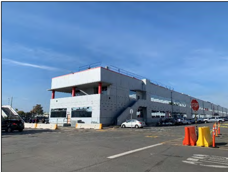
Figure 5.3-6 Building 4, Northeast and Southeast Façades View toward the north.
