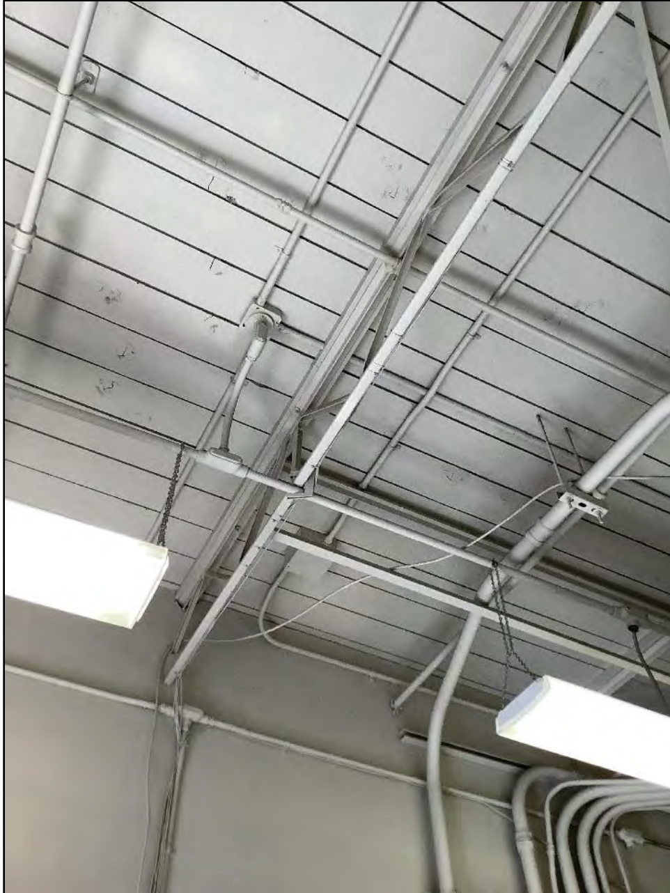
Figure 5.8-3 Ceiling of Building 30
