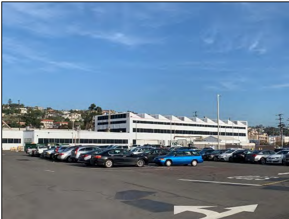
Figure 5.5-1 Building 8, Northwest and Southwest Façades View toward the east.
