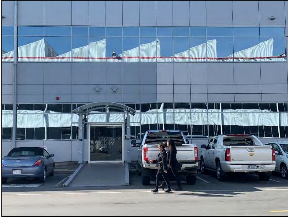
Figure 5.3-9 Building 4, New Entrance at Northeast Façade View toward the southwest.
