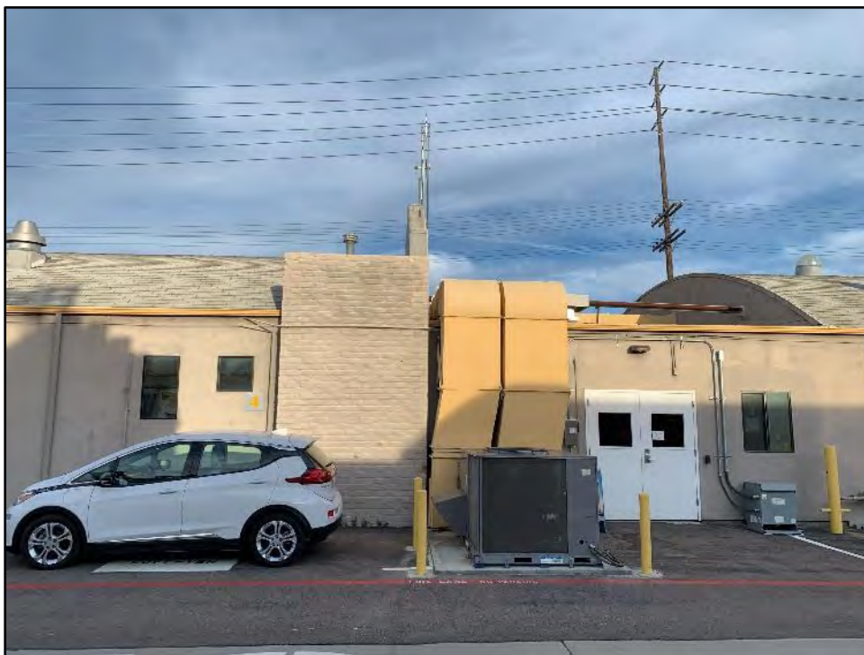
Figure 5.14-29 Detail of the West Façade of Connection between Buildings 4 and 2 View toward the east.
