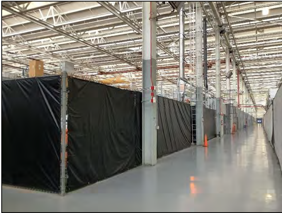
Figure 5.2-34 Building 2 Interior, Corridor with Fenced Storage Areas View toward the east.
