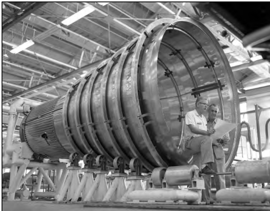
Figure 4.2-27 First Tapered Section Delivered to Building 3 from Plant 71 on Major Assembly Welder September 23, 1960. Courtesy of San Diego Air and Space Museum.
