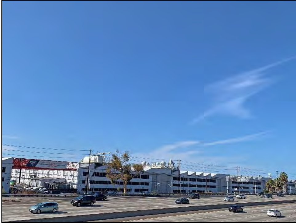
Figure 5.2-24 Building 2, Northeast Façade View toward the west.
