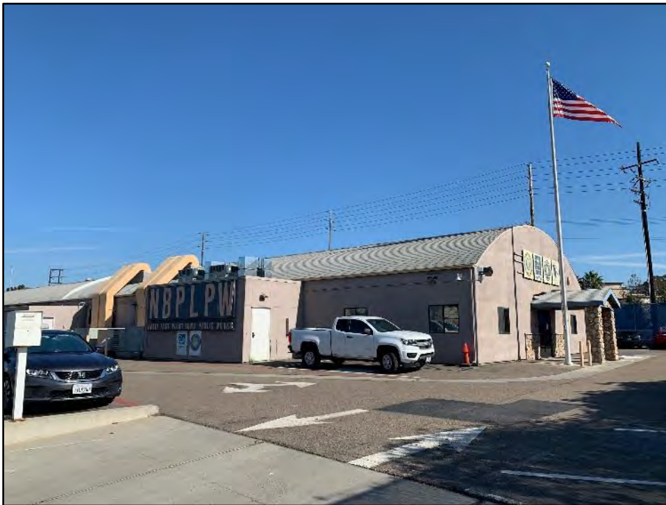
Figure 5.14-13 The West and South Façades of Building 1 View toward the northeast.
