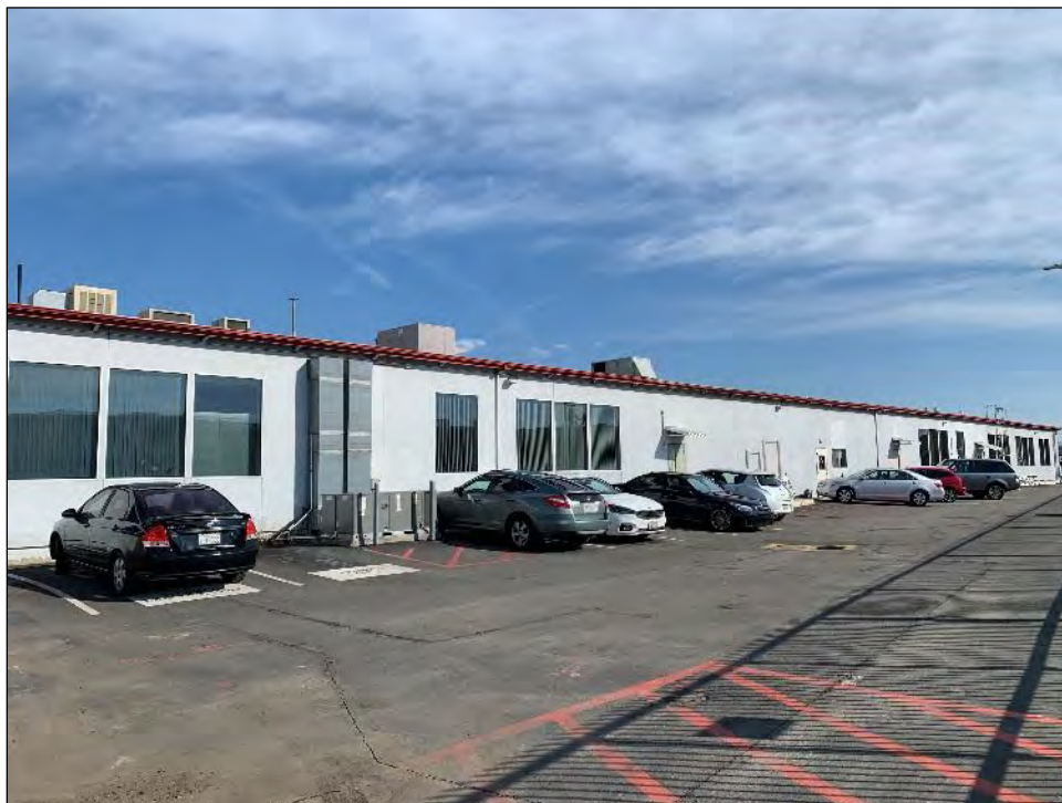
Figure 5.6-2 Building 27, Southwest Façade View toward the east.
