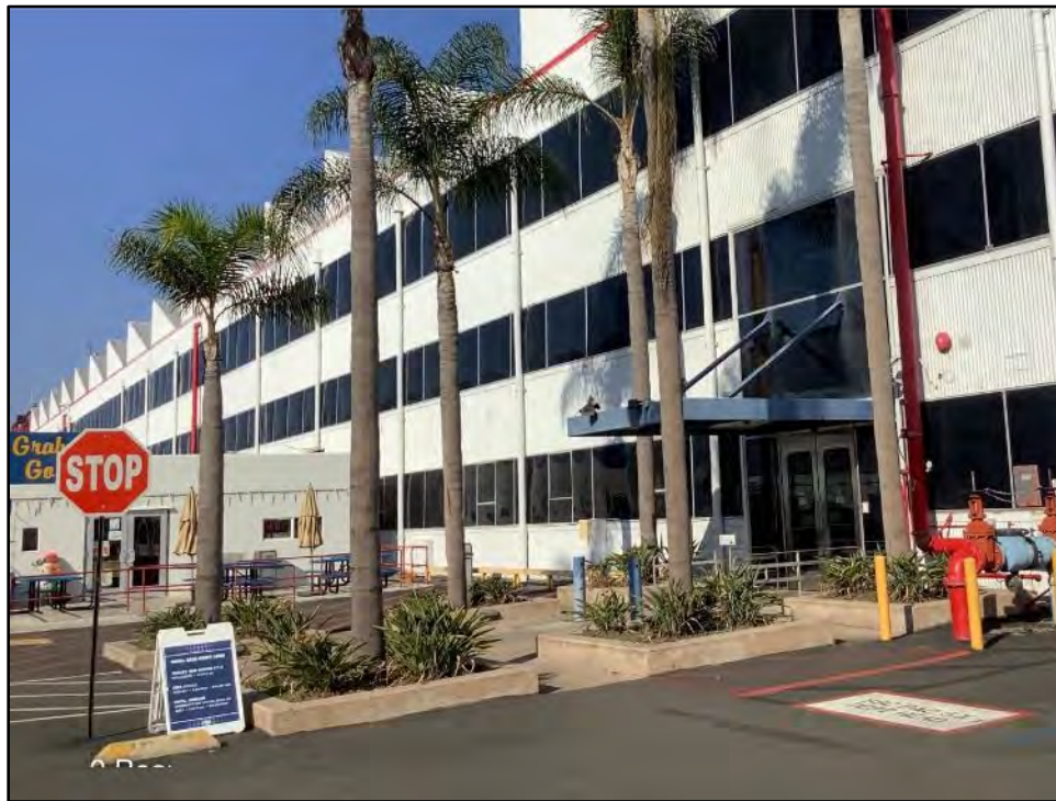
Figure 5.2-26 Building 2, Southwest Façade View toward the north.
