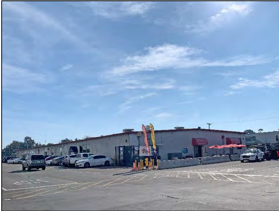
Figure 5.6-1 Building 27, Northwest and Northeast Façades View toward the south.
