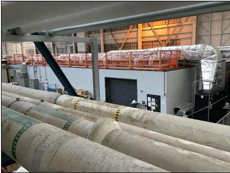
Figure 5.2-31 Building 2, Building within the Main Building View toward the northeast.
