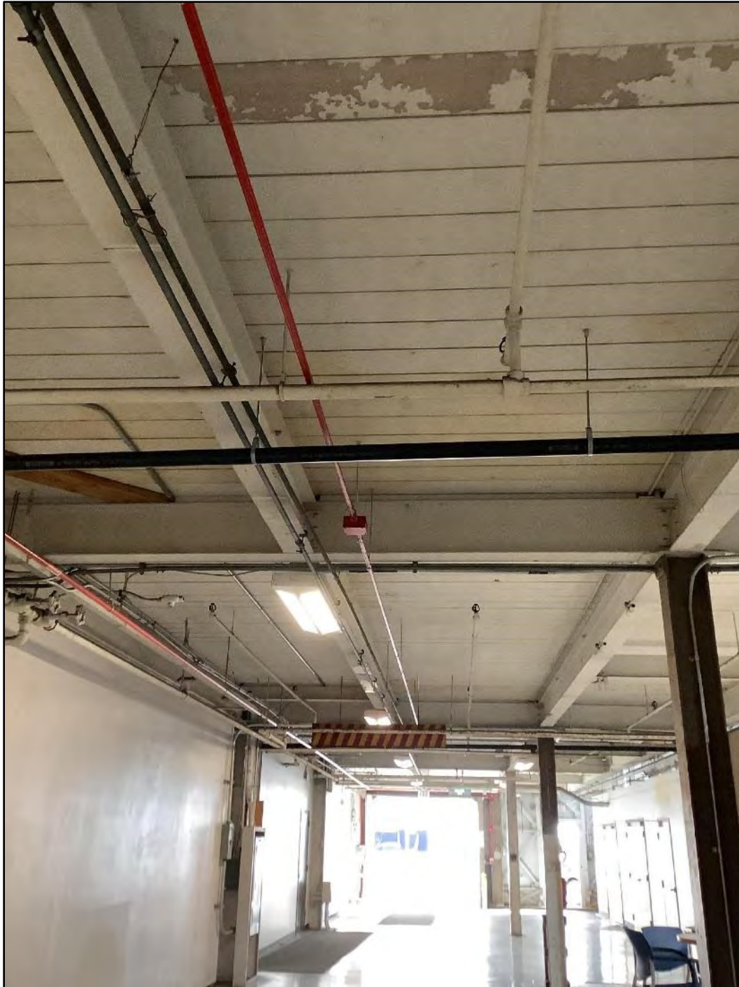
Figure 5.2-19 Building 1 Interior, Wood Board Flooring on Second Floor Mezzanine View toward the southeast.
