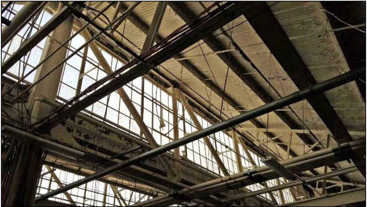
Figure 5.2-44 Building 3 Interior, Showing Sawtooth Windows from the Highest Mezzanine View facing northeast.
