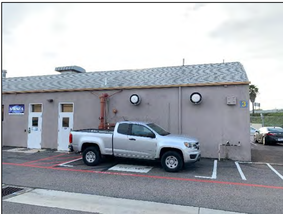
Figure 5.14-23 Detail of the North End of the East Façade of Building 3 View toward the west.
