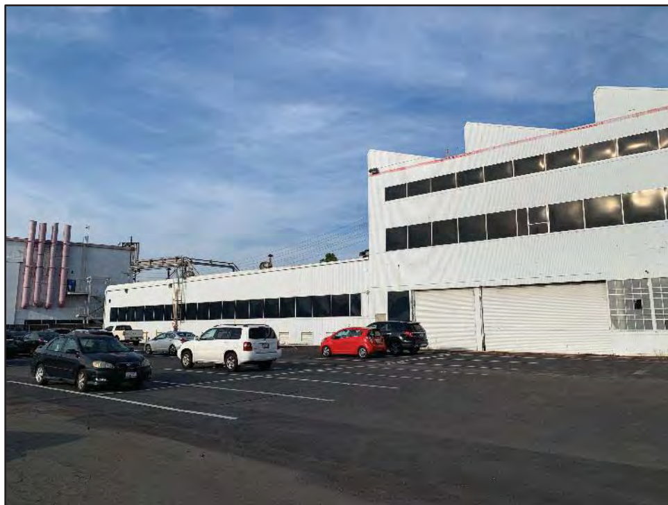
Image 4. Building 8, Northwest End of Southwest Façade. View toward the north.
