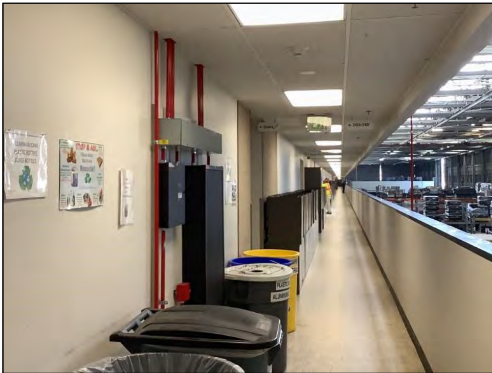
Figure 5.2-23 Building 1 Interior, Mezzanine Corridor View toward the northwest.
