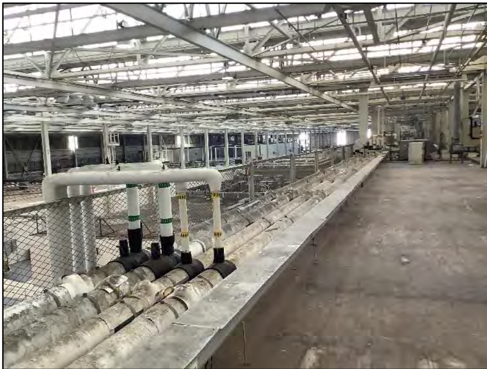
Figure 5.2-15 Building 1 Interior, Third Floor Mezzanine View toward the west.
