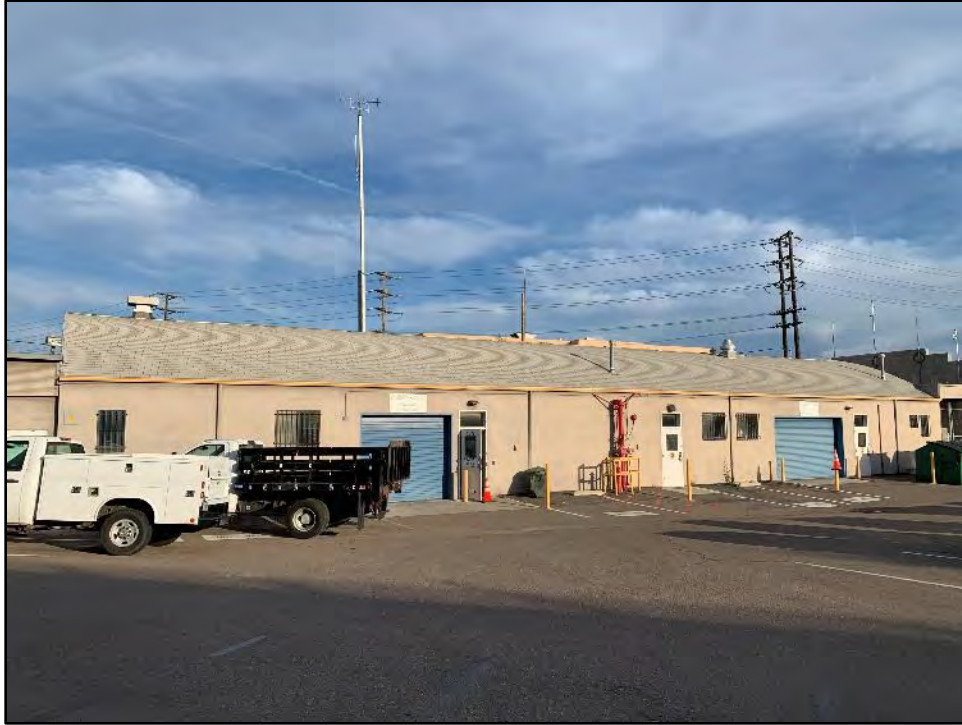
Figure 5.14-26 The West Façade of Building 4 View toward the east.
