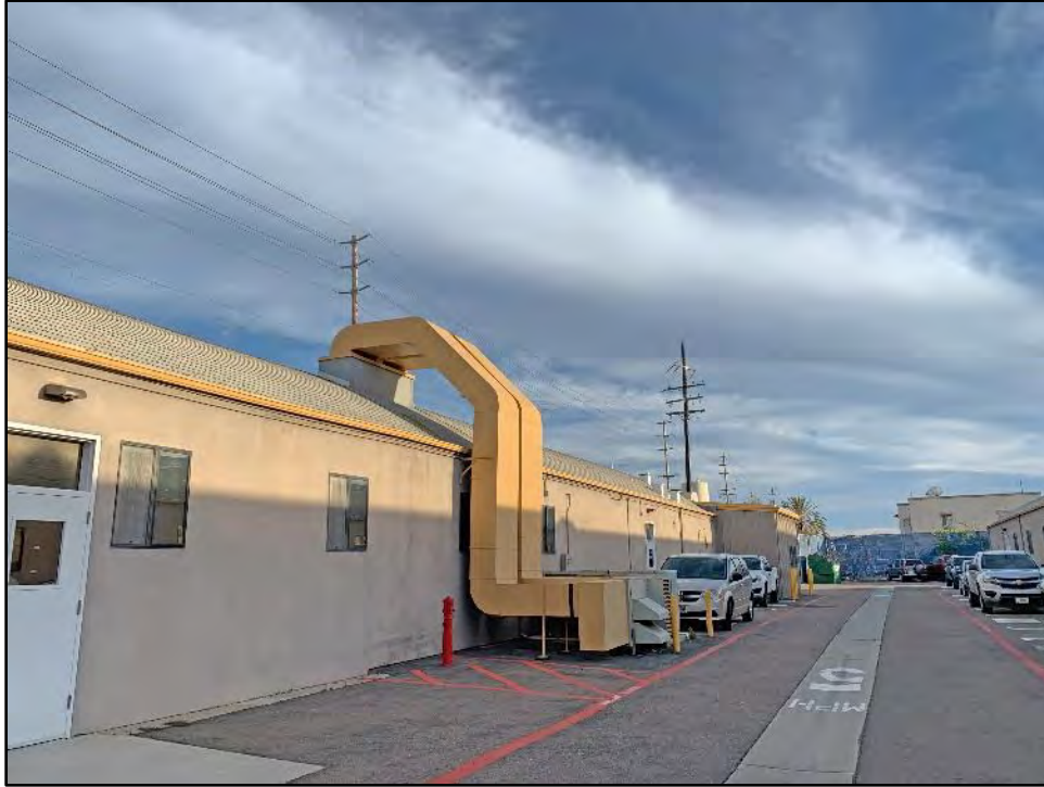
Figure 5.14-20 The West Façade of Building 2 View toward the southeast.
