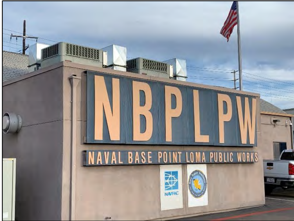
Figure 5.14-18 Detail of the West Façade of Building 1 South View toward the southeast.
