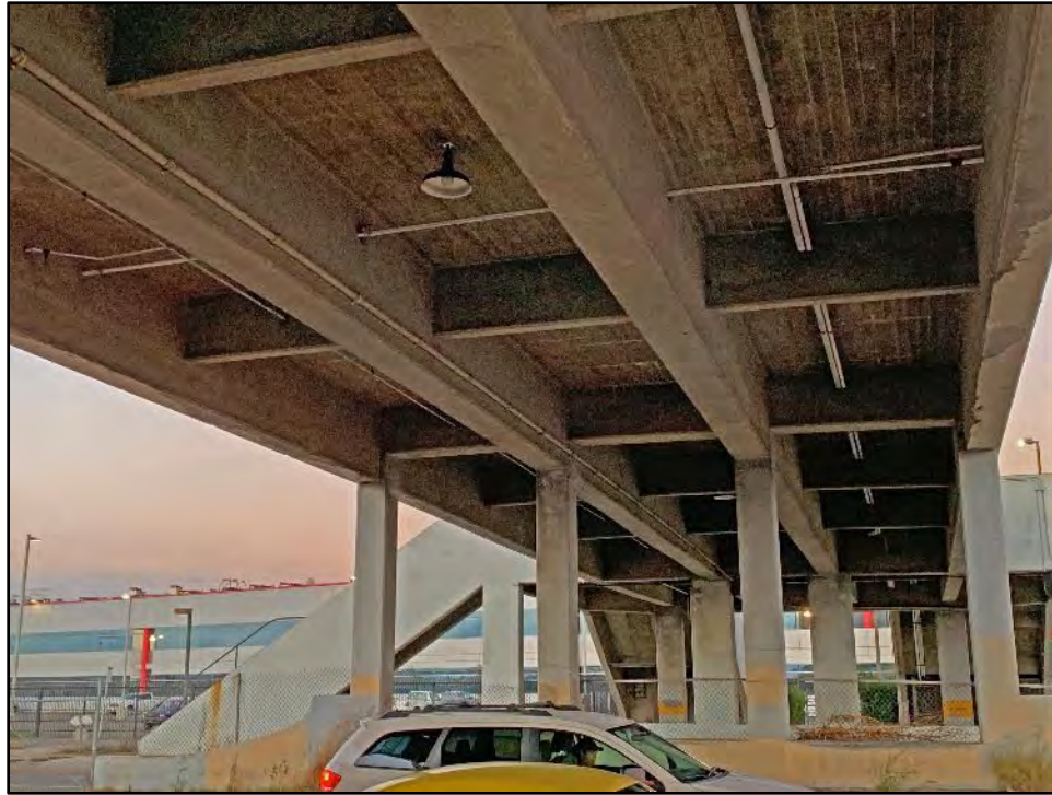
Figure 5.13-9 Detail of the Underside of the Deck View toward the east.
