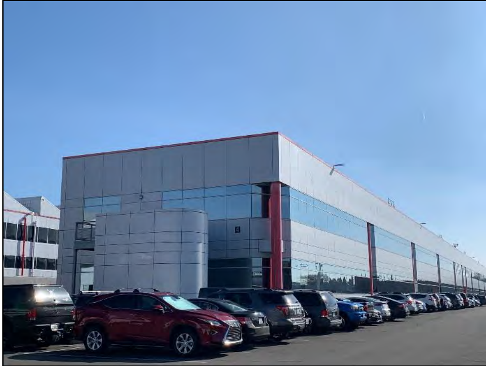
Figure 5.3-5 Building 4, Northwest and Southwest Façades View toward the south.
