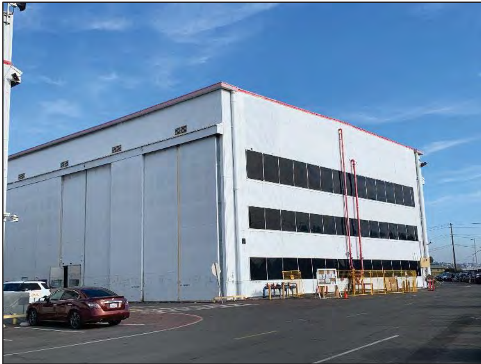
Image 1. Building 7, Northwest and Southwest Façades. View toward the east.
