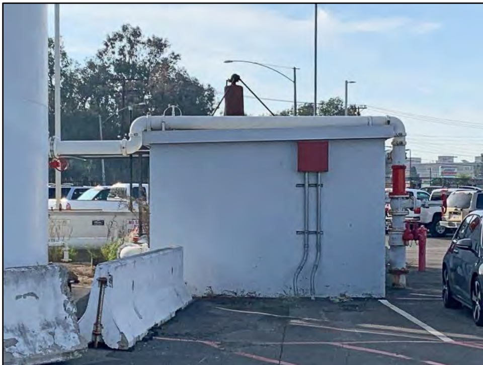
Figure 5.10-3 Building 37, the East Façade View toward the west.
