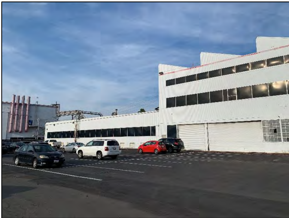
Figure 5.5-5 Building 8, Northwest End of Southwest Façade View toward the north.
