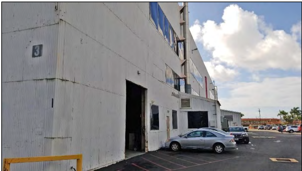
Figure 5.2-42 Building 3, the Northwest Façade View toward the west.
