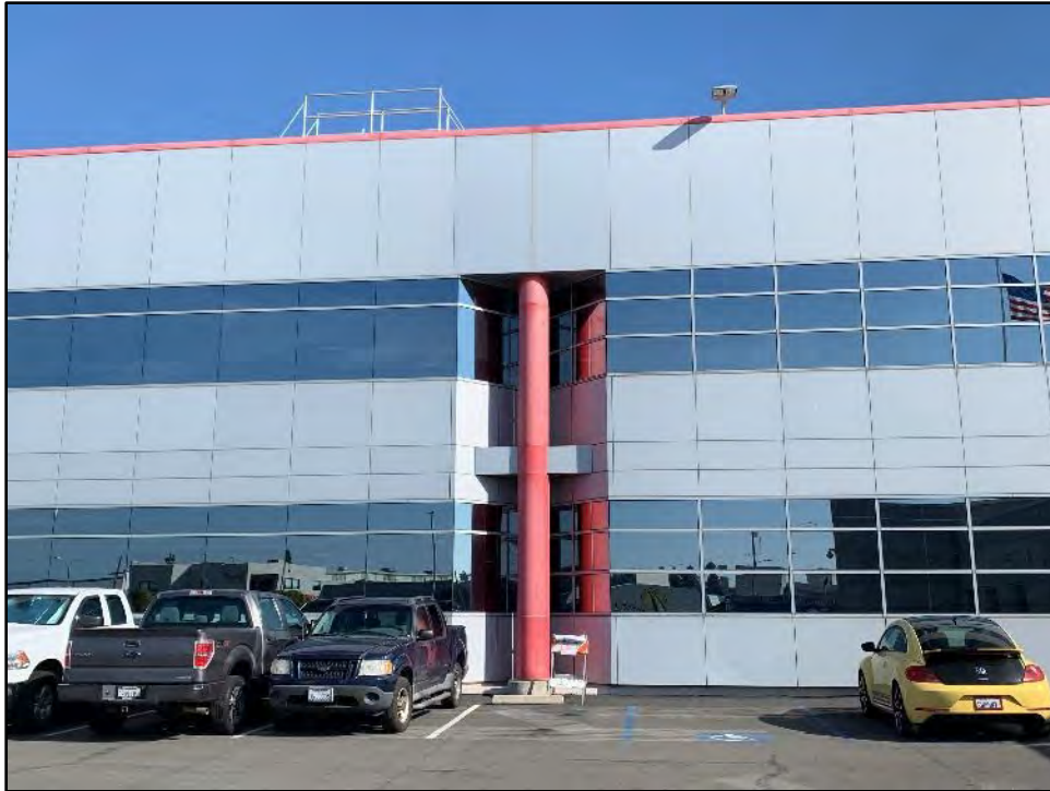
Figure 5.3-7 Building 4, Detail of Southwest Façade View toward the northeast.
