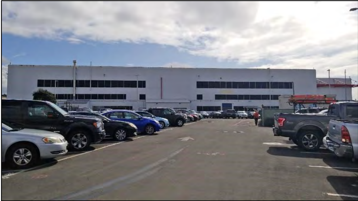
Figure 5.2-40 Building 3, the Northwest Façade View toward the southeast.
