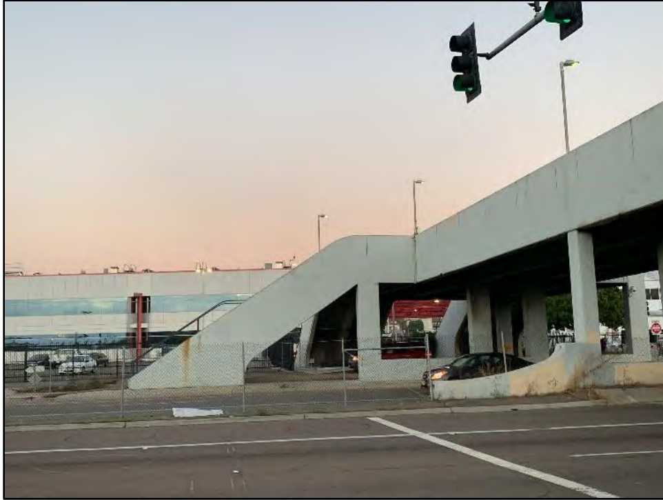
Figure 5.13-7 The Northwest Side of the Bridge View toward the east.
