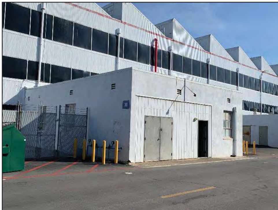
Image 1. Building 30, the Northwest and Southwest Façades. View toward the east.
