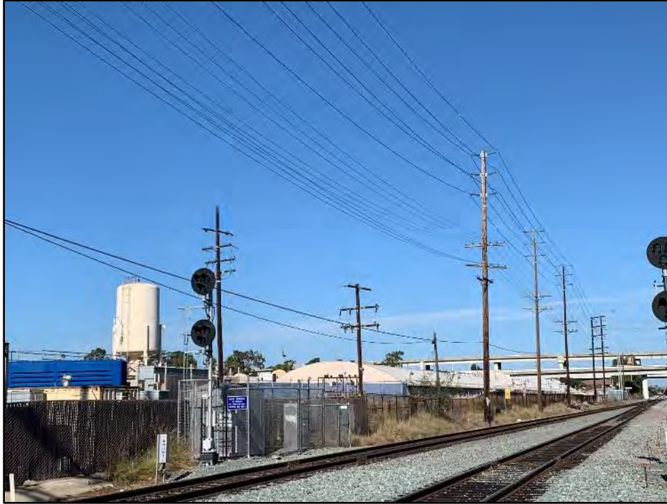
Figure 5.14-10 Overview of the Complex and Railroad Looking toward the Northwest
