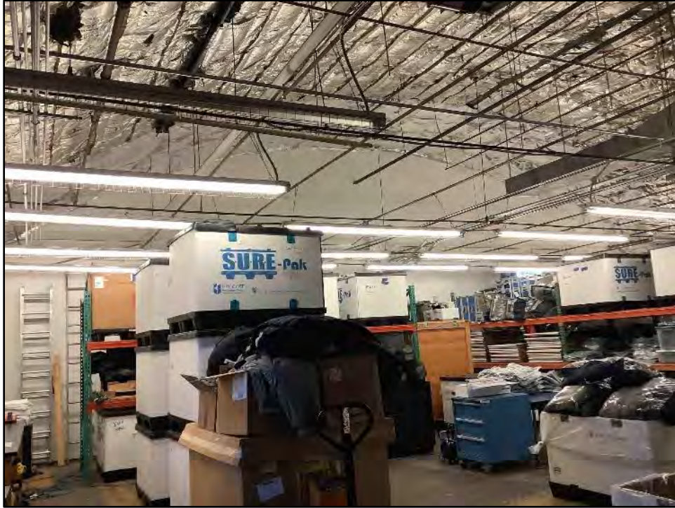
Figure 5.14-40 Storage Area in Building 3 View toward the south.
