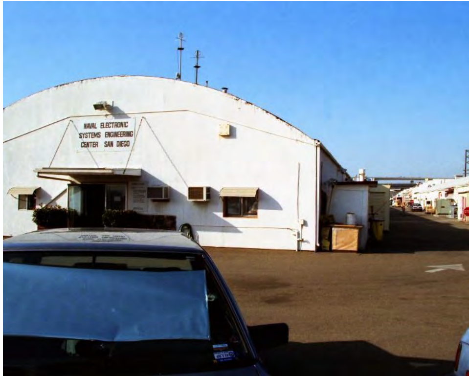
Figure 5.14-12 Historic View of the South Façade of Building 1, undated Source: TSC Tech Library archives.
