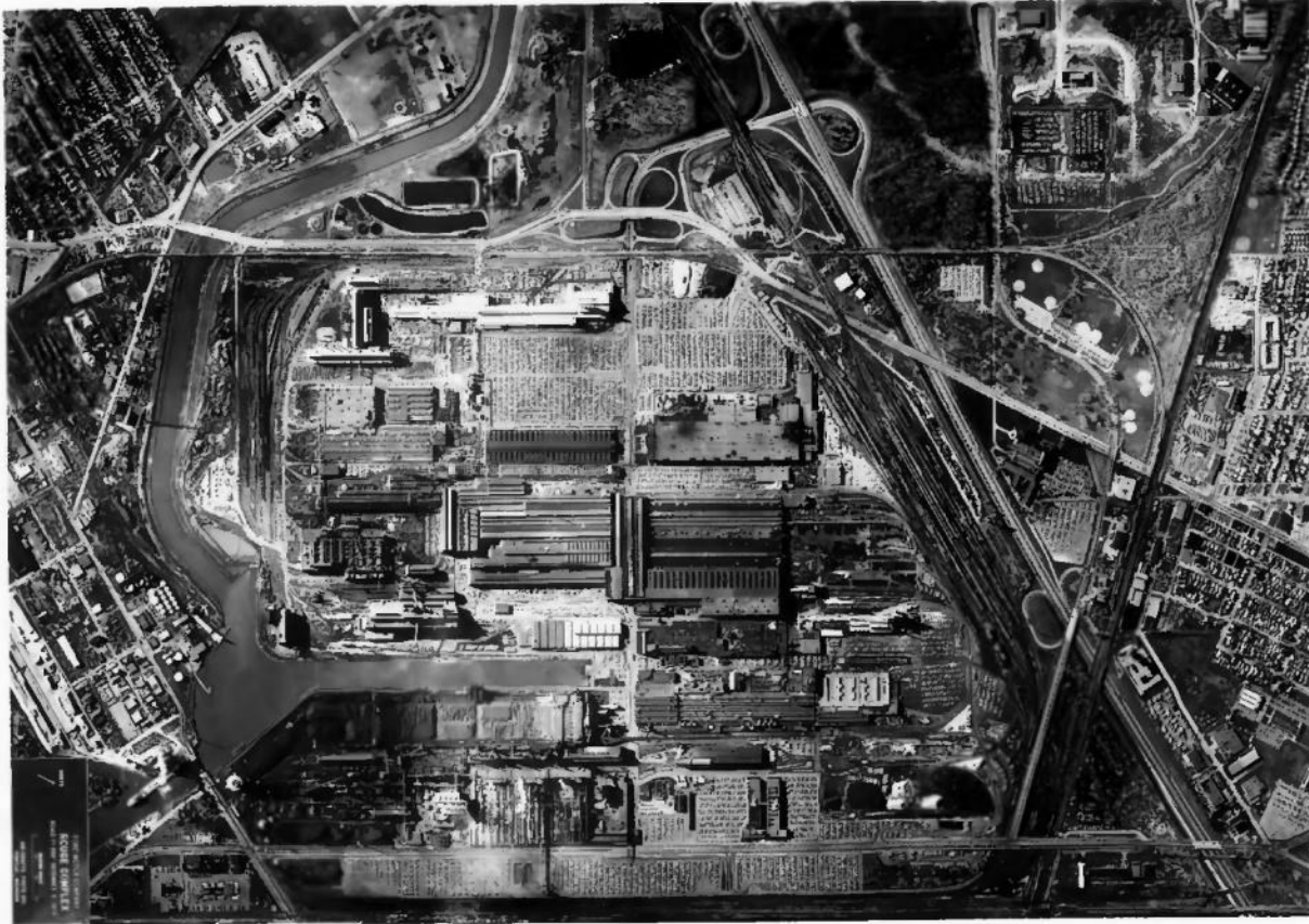
Figure 4.4-4 River Rouge Plant, Ford Motor Company, 1975, Designed by Albert Kahn
