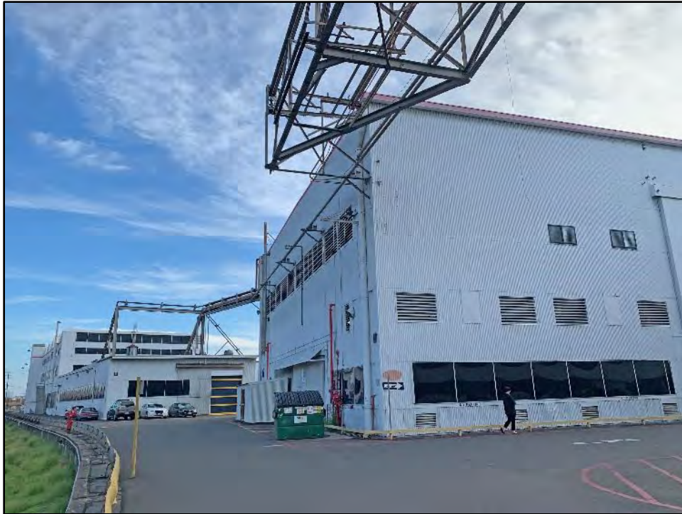
Figure 5.4-5 Building 7, Northwest and Northeast Façades View toward the south.
