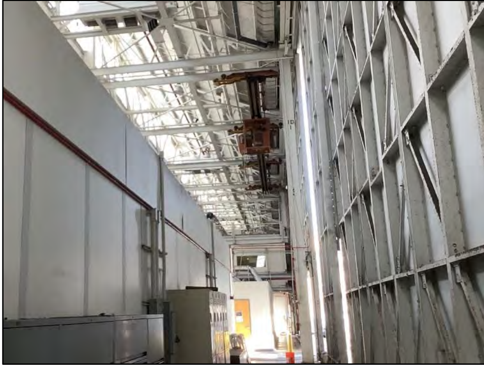
Figure 5.2-8 Building 1 Interior View toward the northeast.
