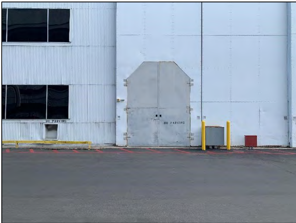
Figure 5.4-4 Building 7, Detail of Door at Southeast Façade. View toward the northwest.
